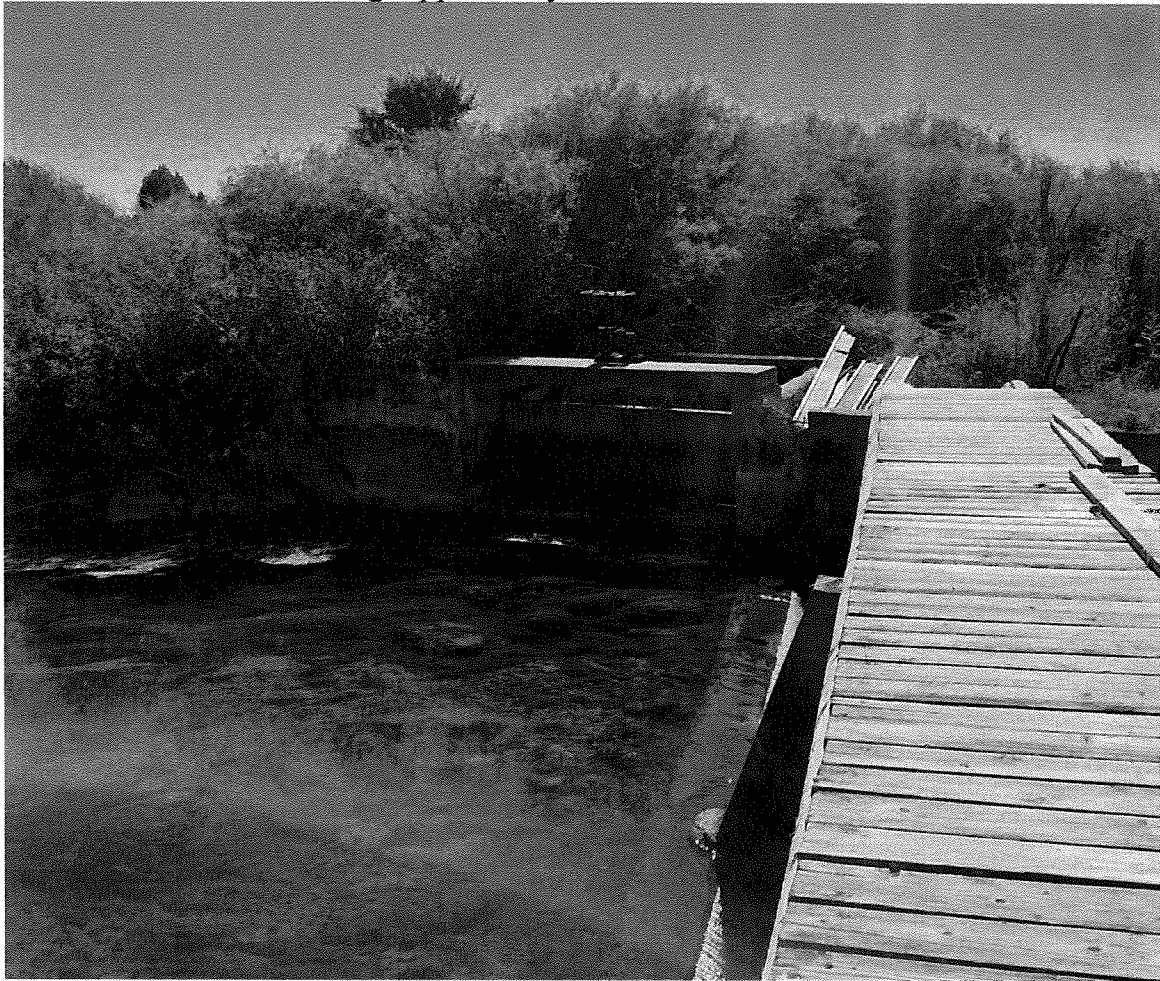
Island Ward Canal Headgate
