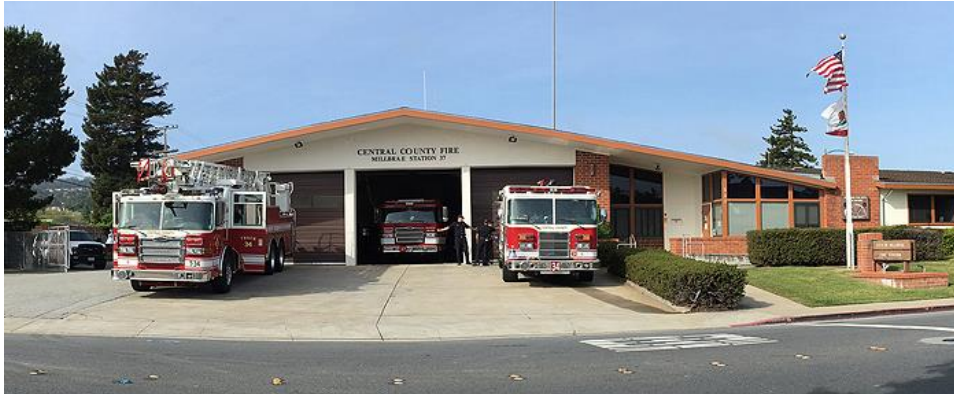
Figure 3: Current City of Millbrae Fire Station landscape.
