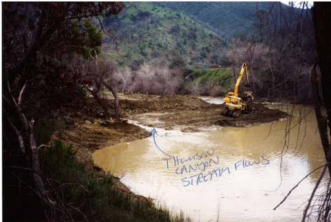
Emergency Excavation of Sediment from Thompson Canyon in 1995
