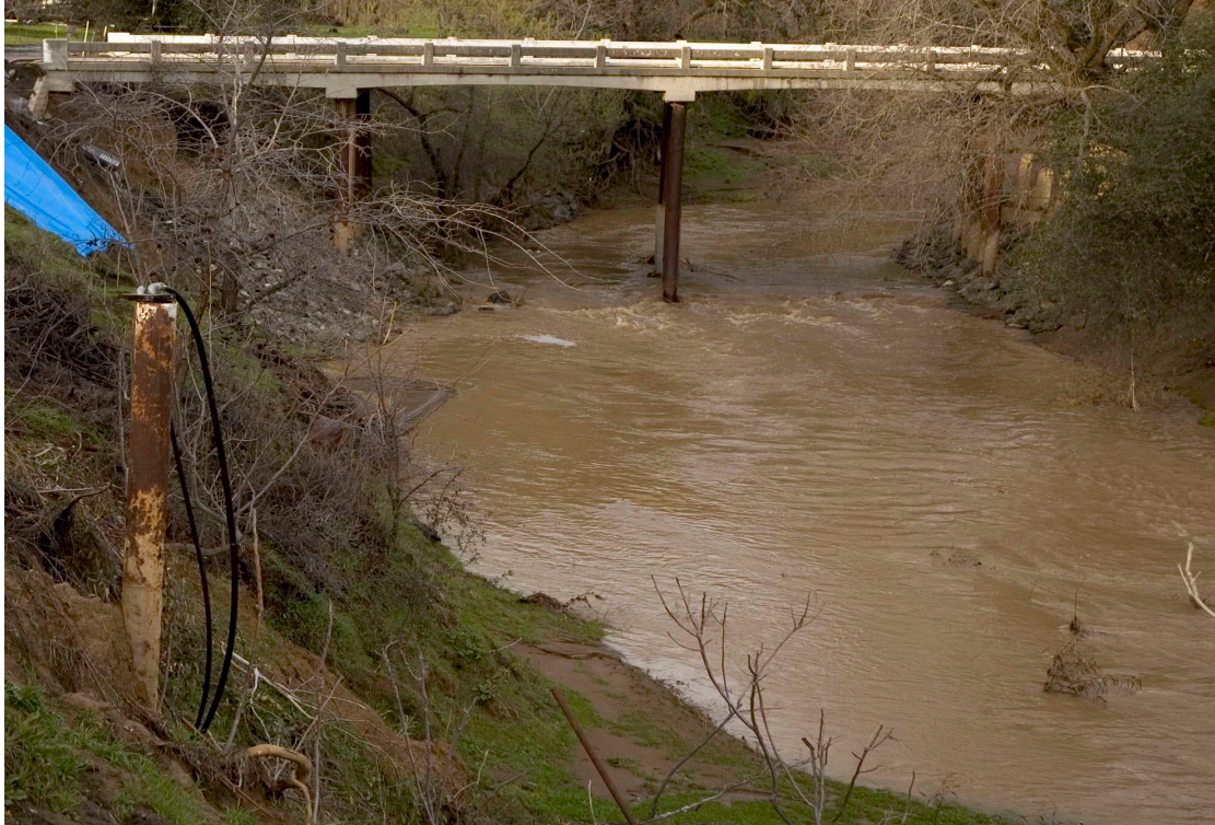
Exposed well casing indicates bank loss on Pleasants Creek (2002)
