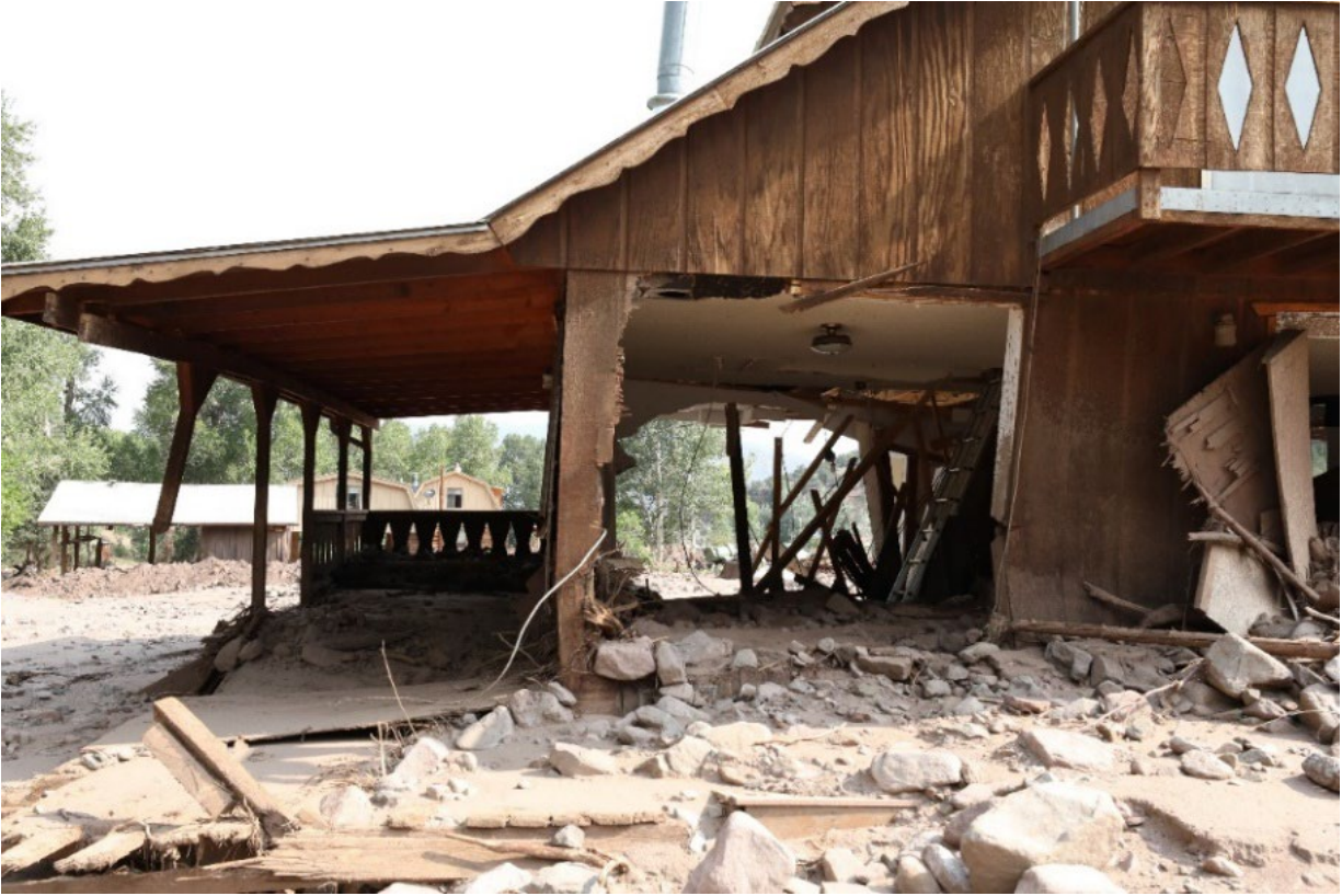
Figure 5. Post-fire flooding damage following Hayden Pass Fire in Fremont County. Photo: ARWC.
