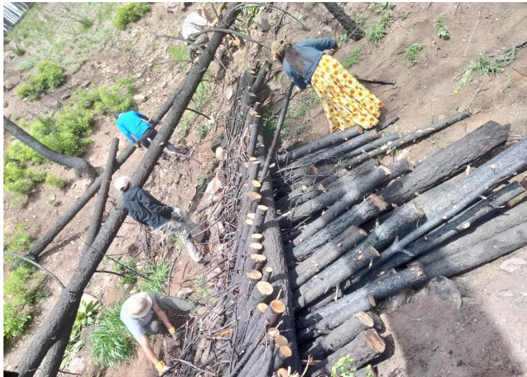
A "trash rack," created in a tributary of the Upper Gallinas River to slow post fire flood waters and sequester sediment. It is an example of one of the many structures used by HPWA to improve watershed quality through the use of available natural materials.
