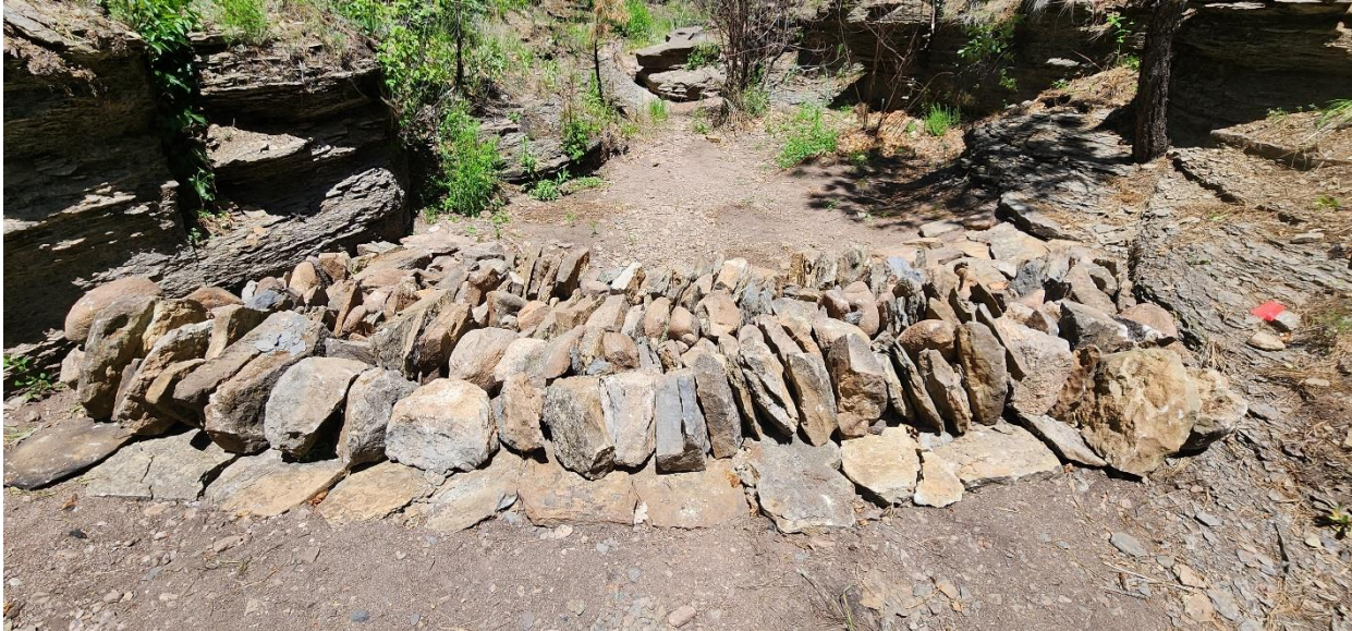
A rock dam constructed to slow water flow near water sources, thereby decreasing or preventing flooding downstream and addressing water erosion.
