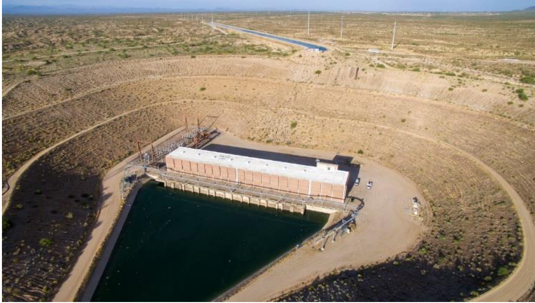
Figure 32. Hassayampa Pumping Plant, one of the 14 pump stations on the CAP's 336 mile-long system (Reclamation photo)
