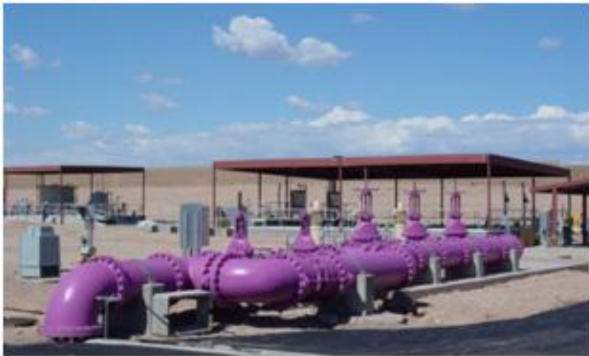
Figure 37. Reclaimed water treatment and distribution site in the study area showing purple pipes. (City of Peoria photo)
