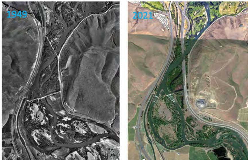
Figure 1-3. 1949 (left) and 2021 (right) aerial photos depicting a left-bank side channel immediately upstream from the Wapato Diversion, which was blocked by freeway bridge construction at the center of the right-hand image.
