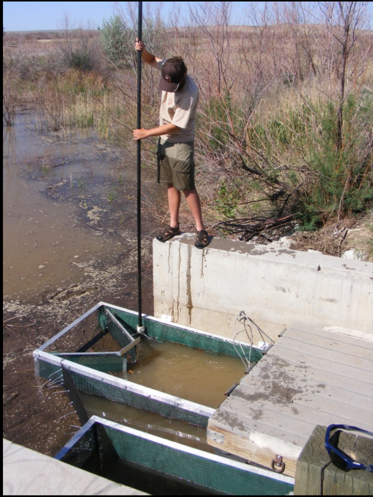
Weir and trap system at outlet gate
