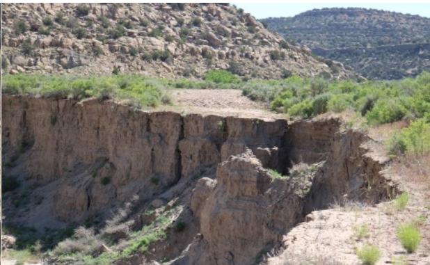
Figure 19 - Previous Bradley Road (completely impassible-eroded by Carrizo Wash)
