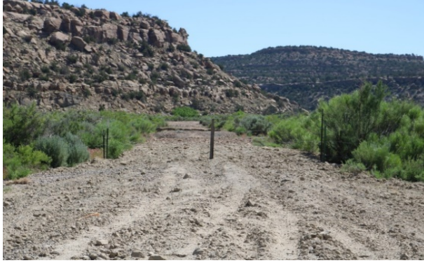
Figure 20 - Previous Bradley Road Ripped and Reseeded with Erosion Control Structure
