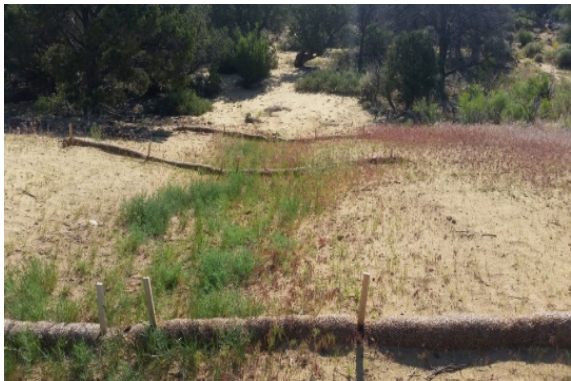
Figure 18 - Recently Installed Silt Trap (Simon Canyon)
