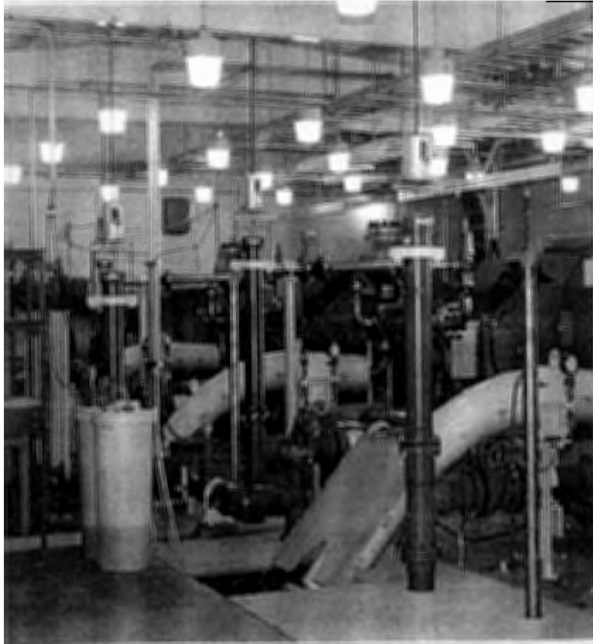
Interior of Brine Injection Facility Three PZ-11 Triplex Positive Displacement Pumps in the Background July 1990 Bureau of Reclamation photo by Tom Wamsley
