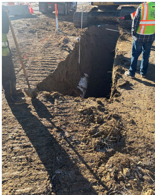
WCA crews exposing Reach 1 to prepare for pipe cleaning and inspection. Reclamation photo
