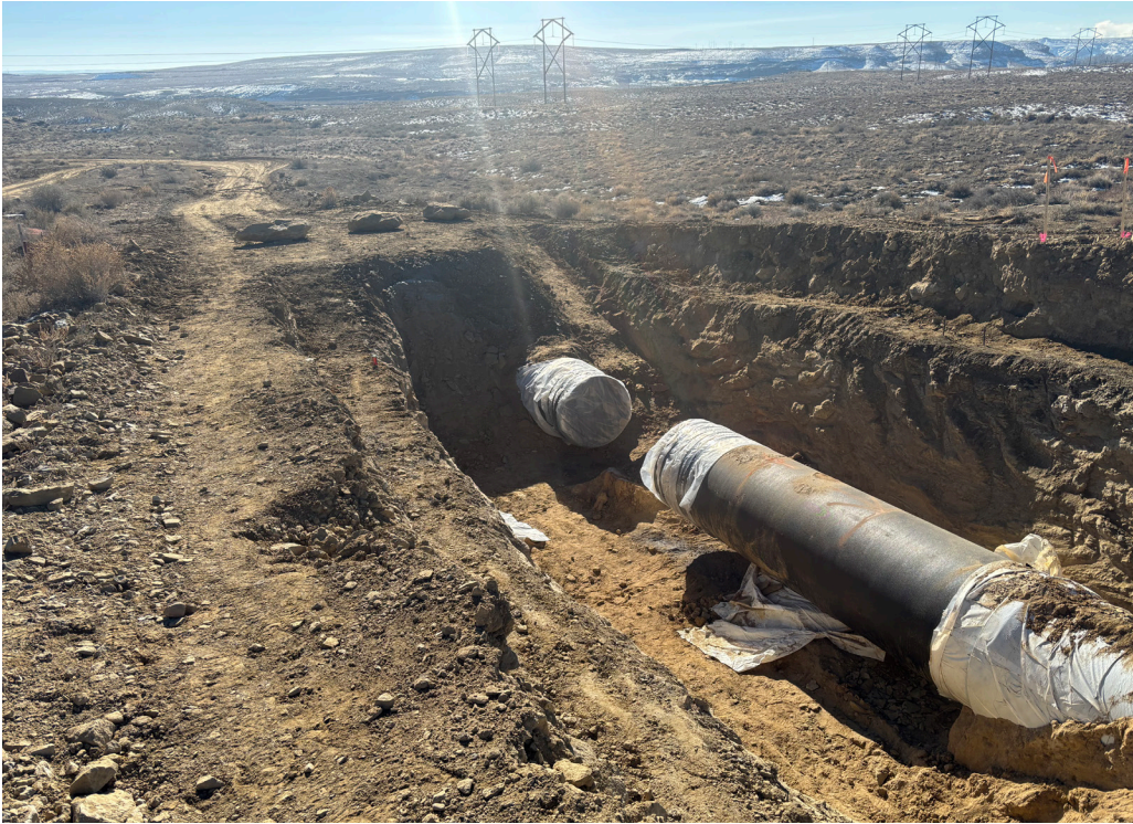
Cut pipe in preparation for pipe cleaning and camera inspection. This is the location of the "T" for the temporary bypass tank. Reclamation photo
