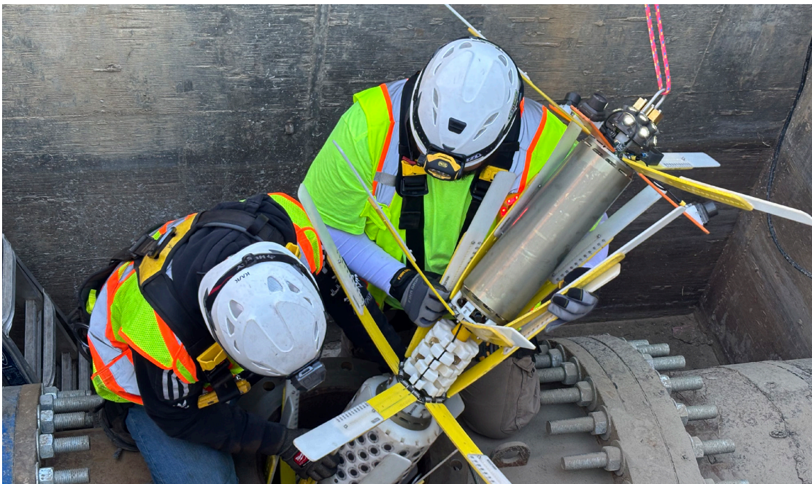
Pipe diver tool being lowered to crew for insertion into Reach 1 pipeline for inspection. Reclamation photo
