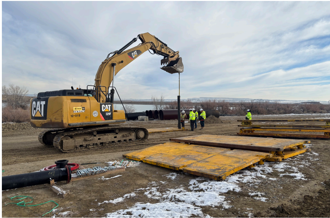
WCA crews assemble trench boxes ready for install. Reclamation photo
