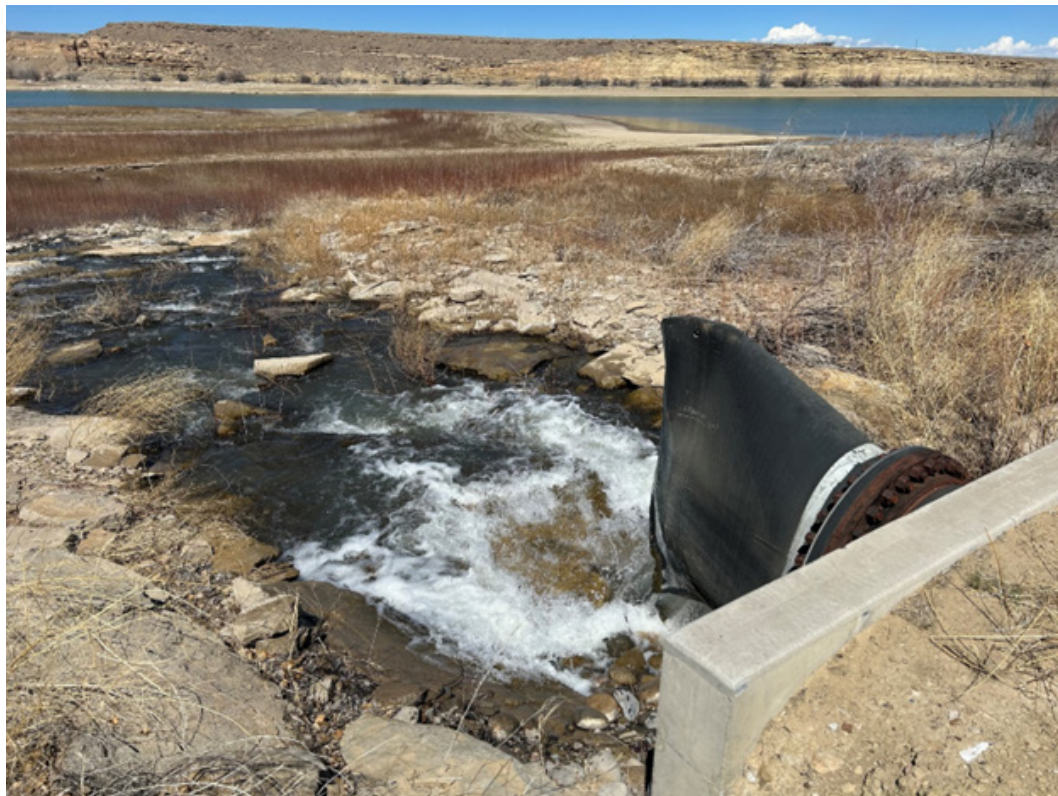
Reach 1 pipeline water discharge location into reservoir (this duckbill valve will be replaced with a flap gate). Reclamation photo
