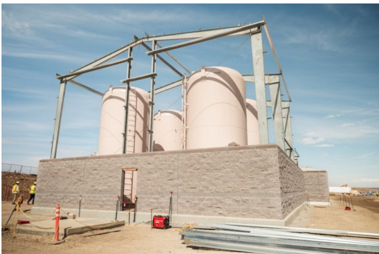
A view of Pumping Plant 3 in progress, showing the four air chambers within the building. Reclamation photo by Pablo Mena
