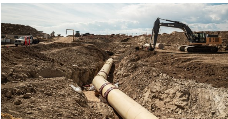
Pipeline construction on the San Juan Lateral near Pumping Plant 3, showing the 42-inch discharge pipeline that will connect to Reach 4C. Reclamation photo by Pablo Mena
