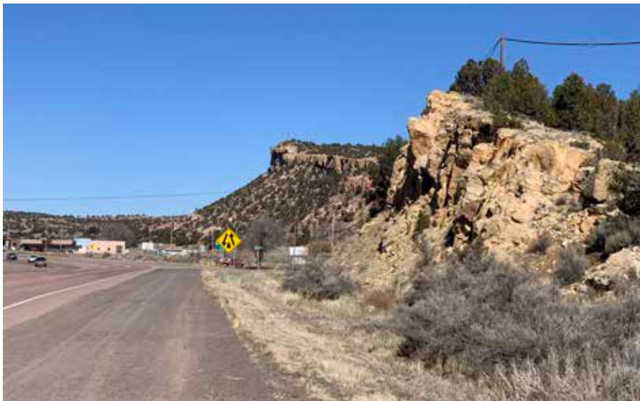
The view looking northwest from NM 264 into Tsé Bonito, New Mexico, where the Code Talkers Lateral will end near the Arizona state line.
