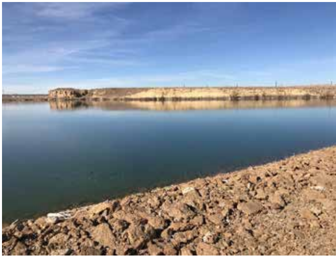
Existing San Juan Generating Station Raw Water Storage Reservoir
