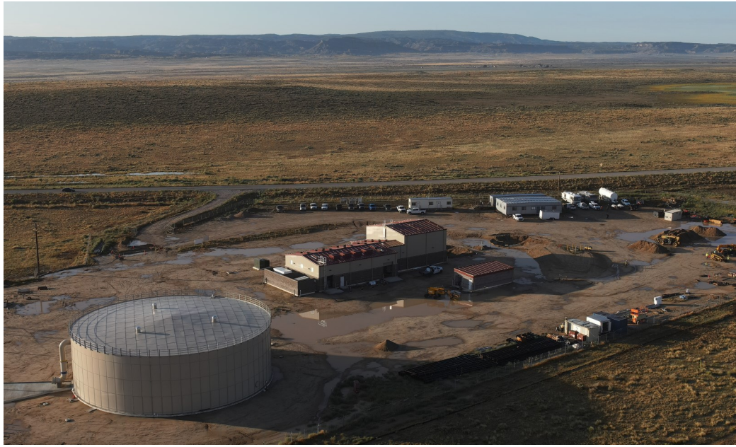
An aerial look of the near finished Bahast'ah Pumping Plant (#7).
