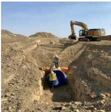
Figure 1 – 42-inch steel pipe installation - Block 4c-8. By Hilda Castillo Smith
