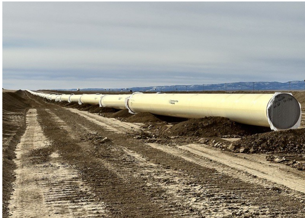
The 42-inch steel pipe ready to be installed on Reaches 4A-4B
