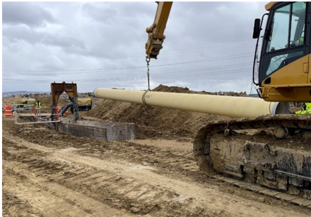
Photo from the Reach 12.1 Construction Site – 30-inch pipeline install
