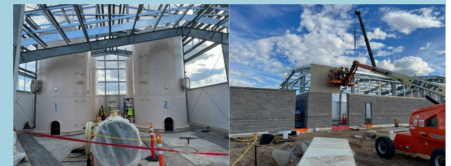
Wall and roof installation at Pumping Plant 7
