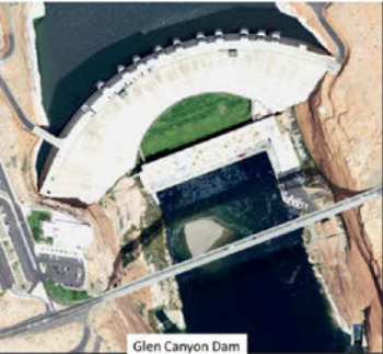
Glen Canyon Dam
