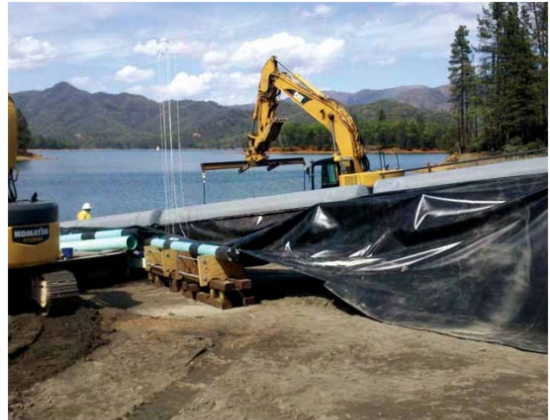
FIGURE 7 The floats and the curtain were deployed using a conveyor system
