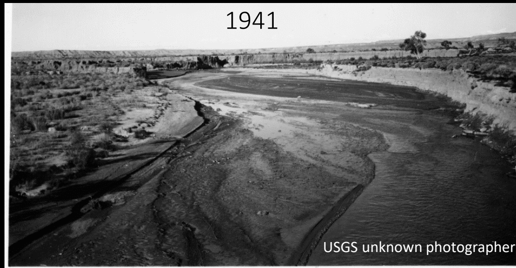
Moenkopi Wash, AZ, Looking upstream from Hwy 89 bridge Near Cameron, AZ
