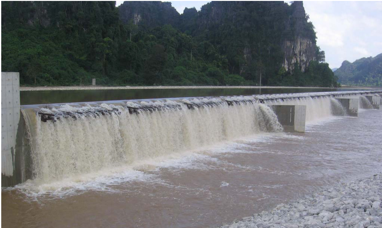
Figure 6.—Picture of an aerating weir in the downstream channel of the regulating dam in the Nam Kathang River (Descoux 2015).
