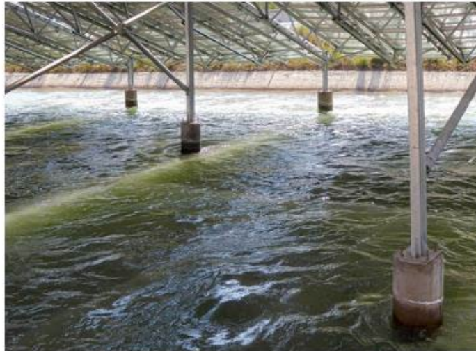
P4P in-canal solar structure providing shade, Punjab, India
