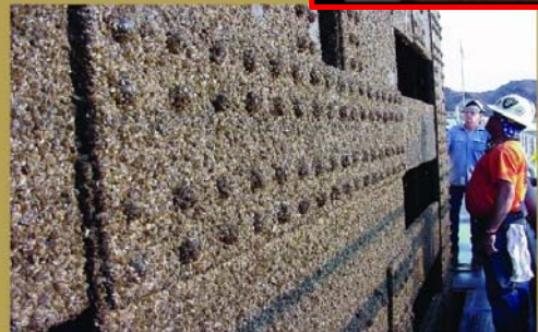
Lake Havasu RECLAMATION
