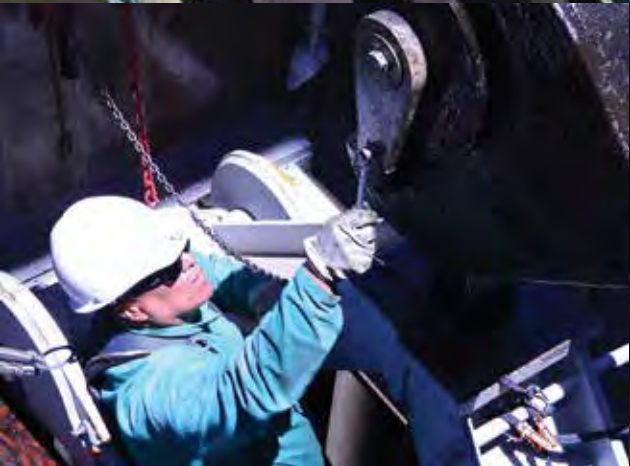
Working on a penstock gate at Glen Canyon Dam, Arizona (Reclamation photo by Chris Watt) BACKGROUND PHOTO: Reclamation officials inspect Lemon Dam, Colorado. (Reclamation photo)
