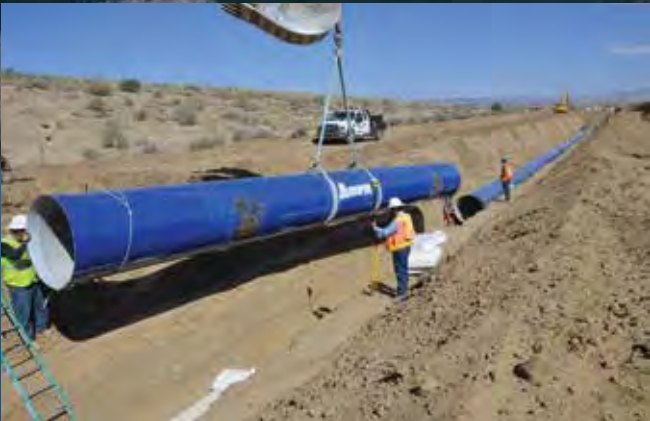
Placement of pipe on Navajo-Gallup Water Supply Project (Reclamation photo)
