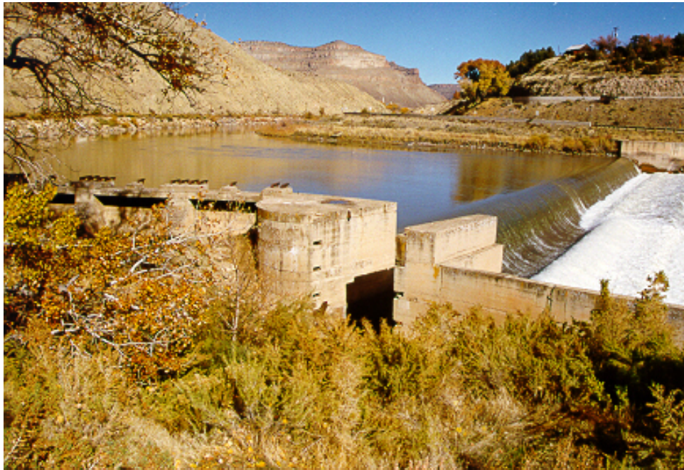
Figure 1—Price-Stubb Diversion Dam on the Colorado River near Palisade, Colorado
