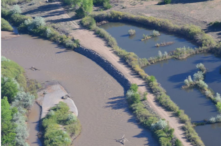
Figure 5: Photo looking north toward completed bank stabilization work at Ohkay Owingeh Pueblo (Reclamation, 2024)
