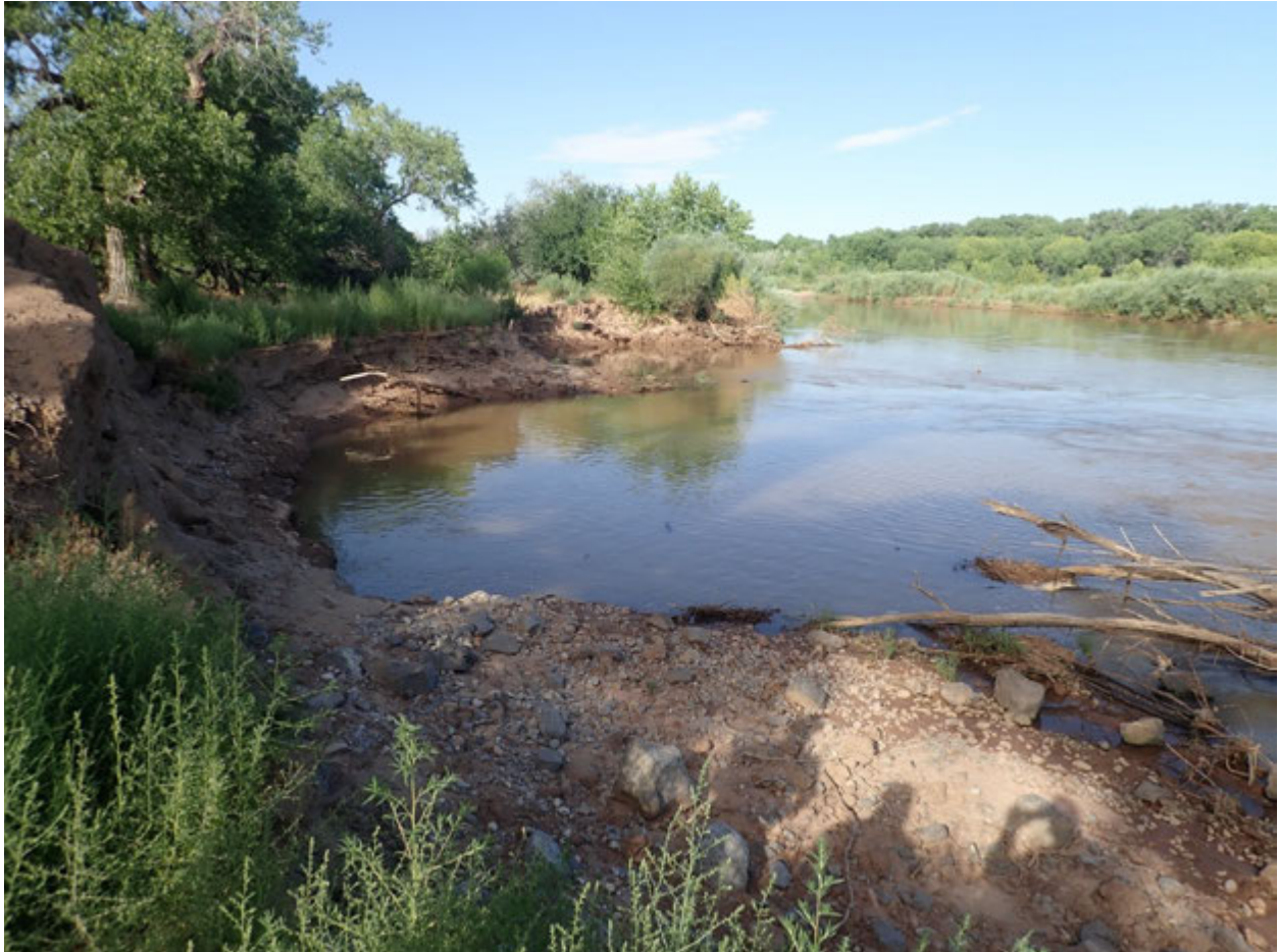
Photo 1: Looking downstream at Santa Ana River Mile 205.8 east bankline bendway weirs and bankline repairs (Reclamation photo)
