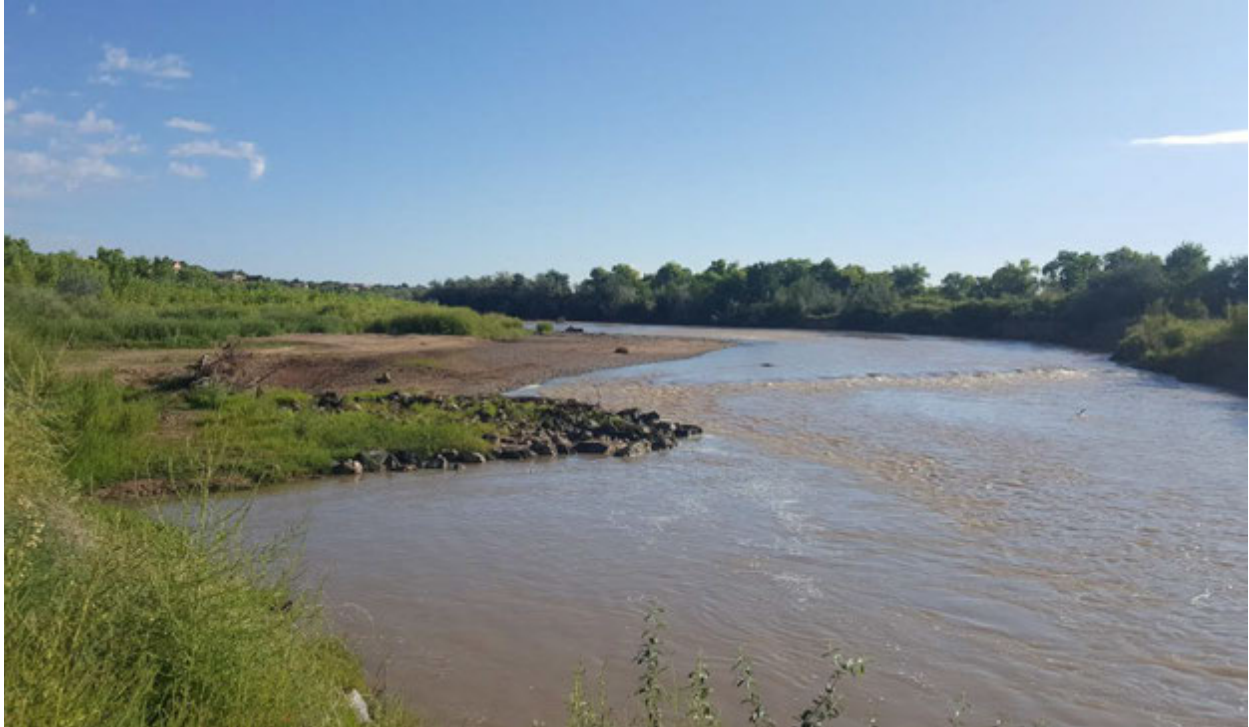
Photo 2: Looking upstream at the Corrales Siphon and the 2016 riprap protection placed downstream of the siphon. The river upstream of the riprap protection has filled in with sediment. (9/11/2019)
