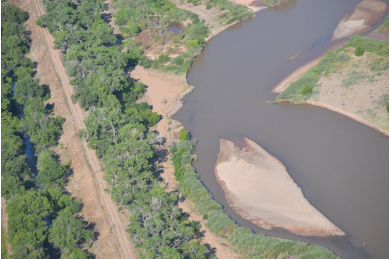
Photo 1: Aerial view of the Sandia Priority Site (flow direction from bottom to top of photo). The eroding bend apex has moved downstream roughly 400 feet in four years and point bar deposition now protects the bankline at the bendway weirs at low flows. (7/18/2019)
