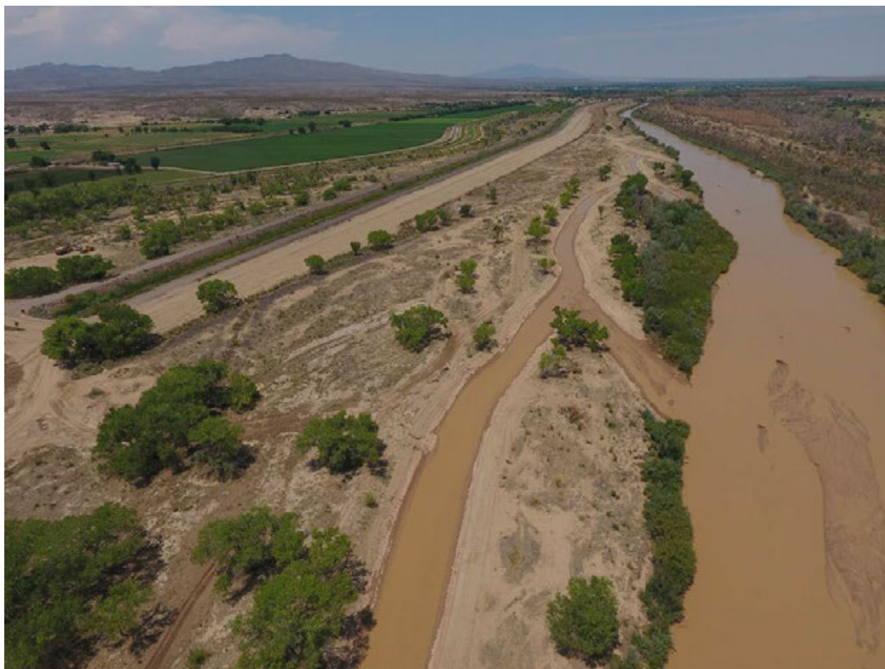
Photo 4: Escondida side channel project at post-monsoonal conditions (7/30/2018)
