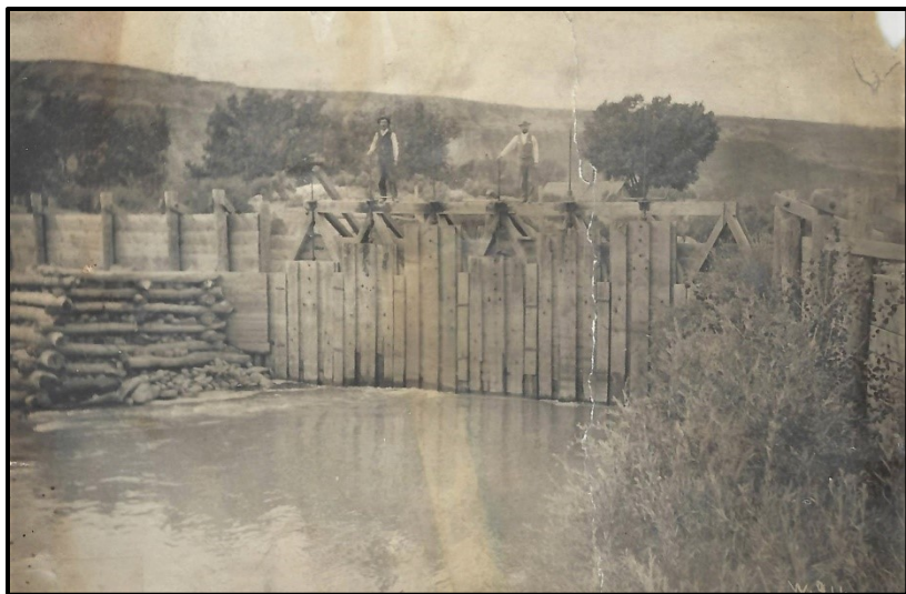
The original headgate for the Grand River Ditch constructed in 1883 (on file at the GVIC, Grand Junction).
