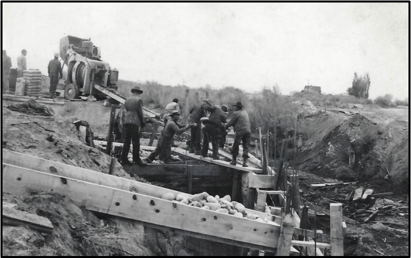
Replacement work underway of Highline Lateral Flume No. 10 across Little Salt Wash, in 1947 (on file at the GVIC, Grand Junction).
