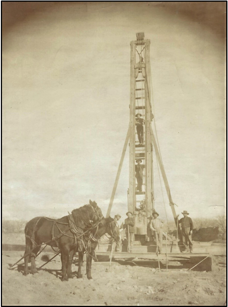
A pile driver is used to construct flumes along the canal routes (on file at the GVIC, Grand Junction).
