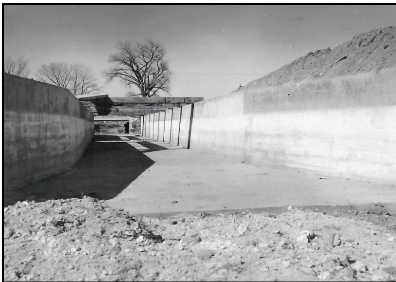
Newly completed concrete Rice Flume at Carpenter Wash on the Main Line in 1956 (on file at the GVIC, Grand Junction).
