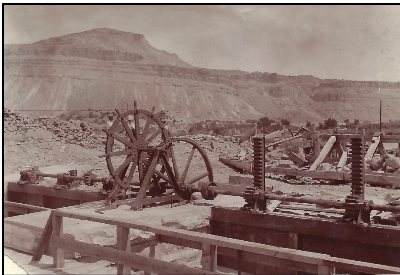
Detail of the gate lifting mechanism of the Grand River Ditch headgate upon completion in 1900 (on file at the GVIC, Grand Junction).
