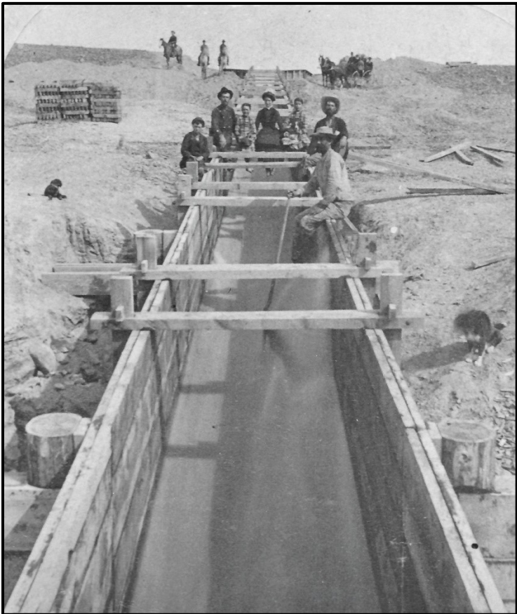
A wooden flume conveys water down the big drop below the division of the Highline and Mainline laterals of the Grand River Ditch about 1883 (on file at the GVIC, Grand Junction).
