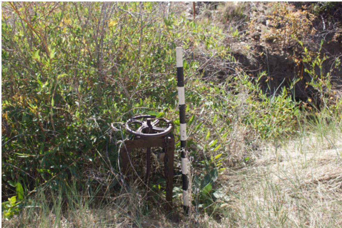
Image Number 5667 A photograph showing a closeup of Feature 4, the Rattliff and Root irrigation ditch lateral headgate's north elevation, facing south.
