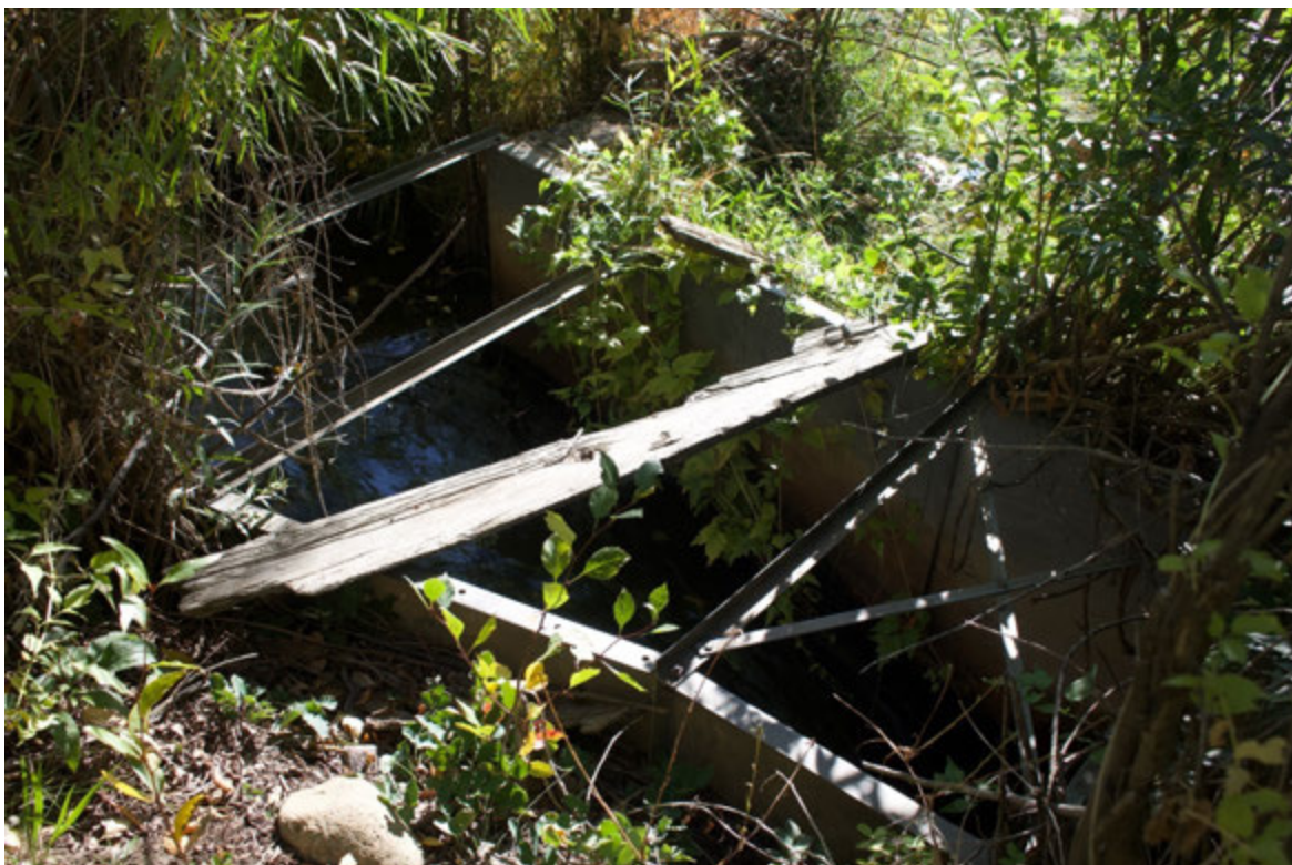
Image 5654 A photograph showing a closeup of Feature 3, the Ratliff and Root irrigation ditch Parshall Flume with lumber laying across top and utilized as a footbridge, facing southeast.
