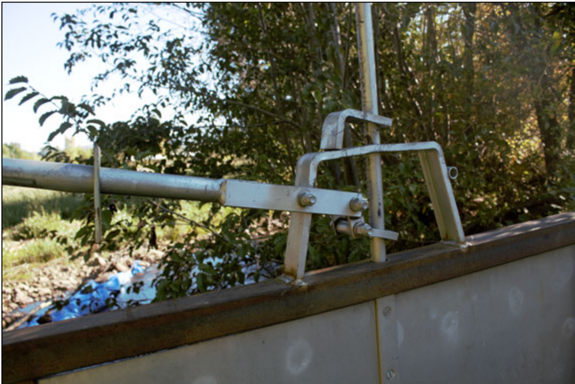
Figure 18. Closeup of the gate lever system in Feature 1. View to the northeast.
