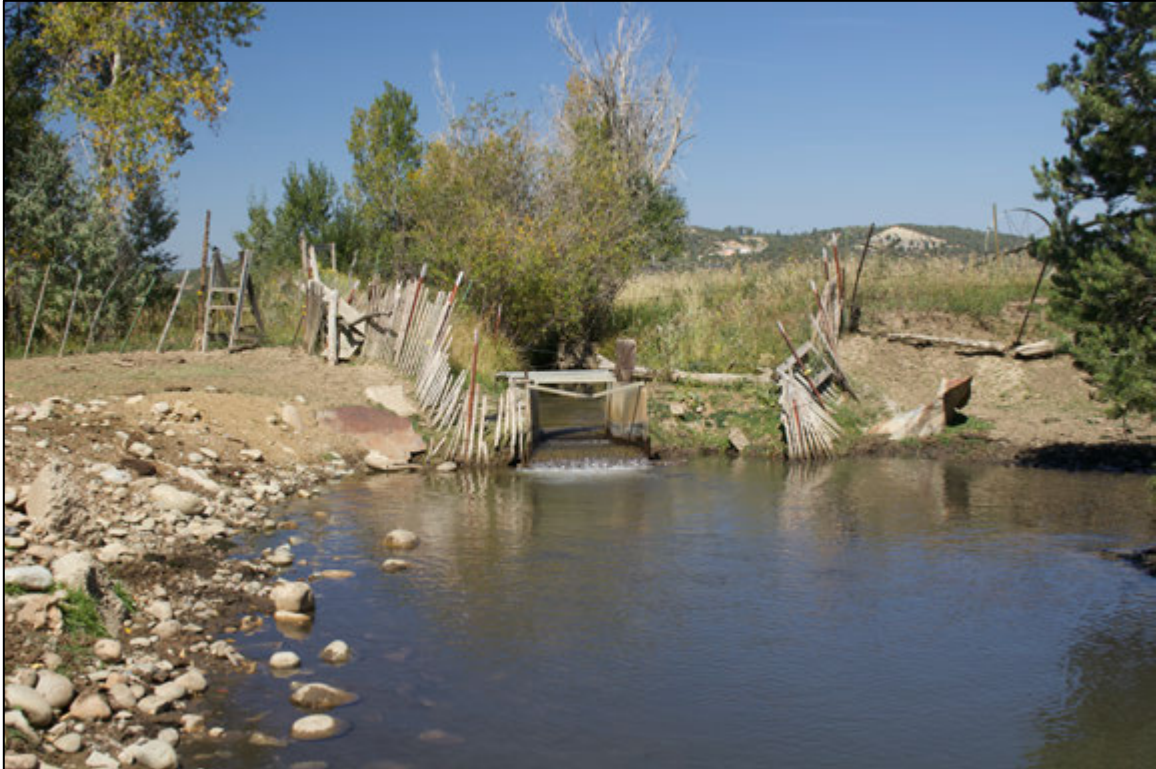
Figure 30. Overview of the Parshall Flume in Feature 5 facing north.
