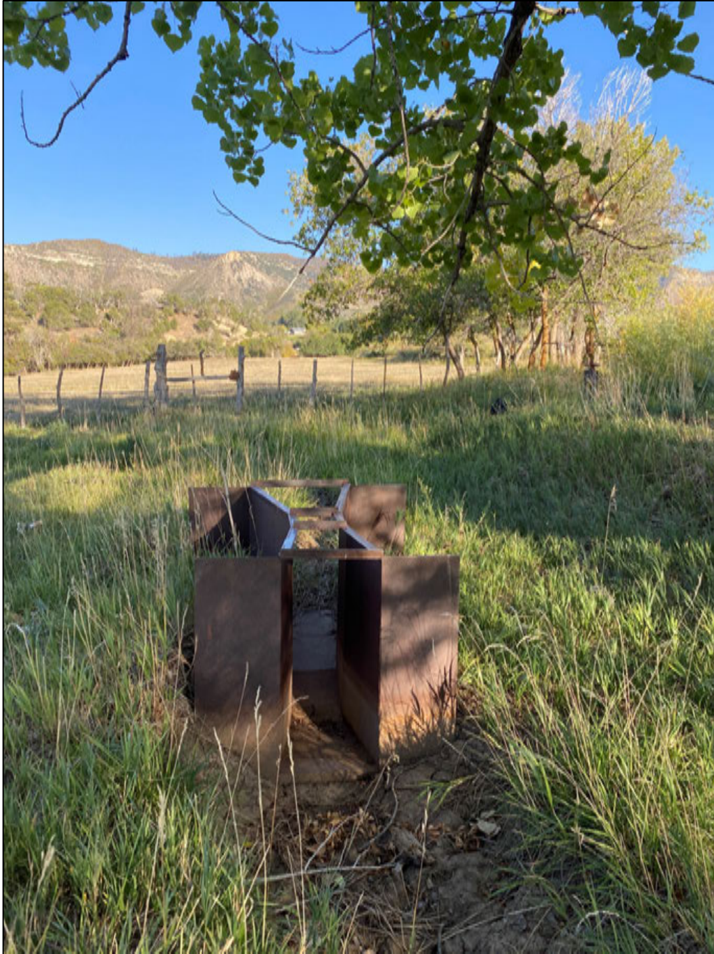
Figure 42. Closeup of the Parshall Flume in Figure 9.
