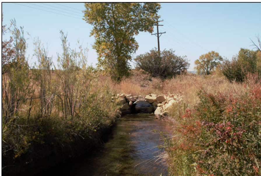
Figure 14. Example of a modern 2 foot in diameter corrugated metal culvert along the Ratliff and Root Ditch.
