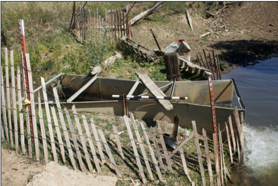
Figure 31. Overview of the Parshall Flume in Feature 5 facing east.
