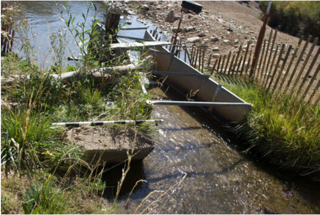
Image Number 5682 A photograph showing a closeup of Feature 5, the Ratliff and Root irrigation ditch Parshall Flume No. 2, facing southeast.
