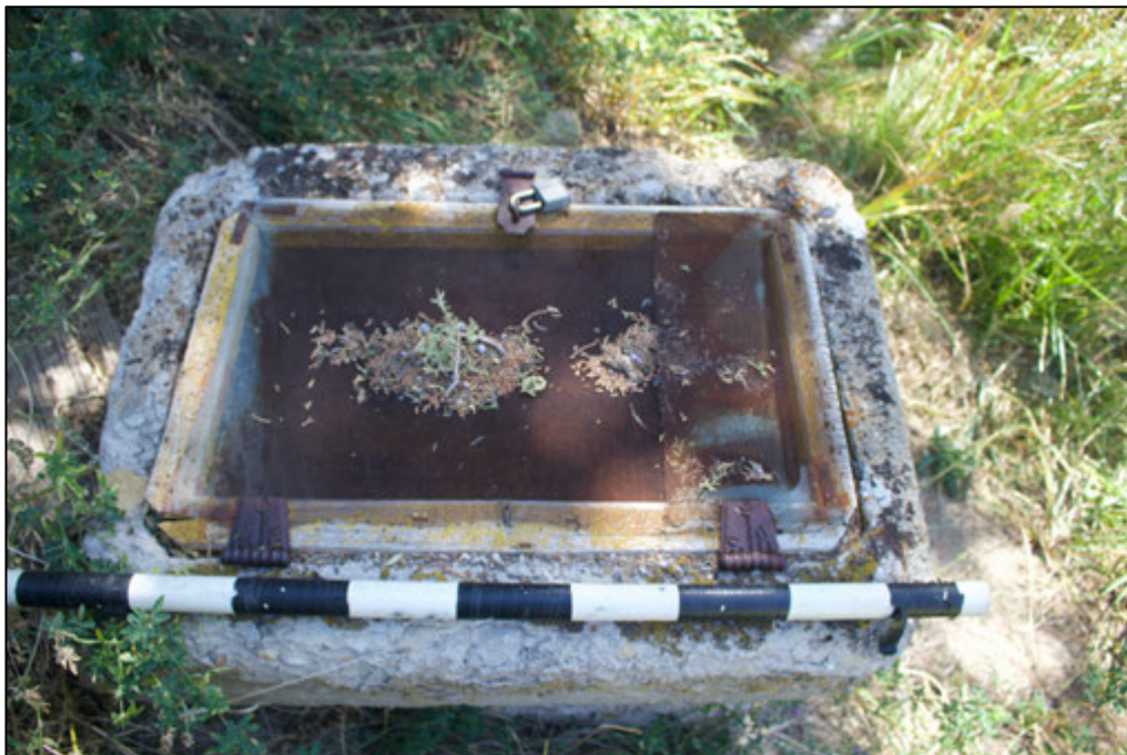
Figure 37. Closeup of the hinged screen over the stilling well in Feature 7. View to the southwest.
