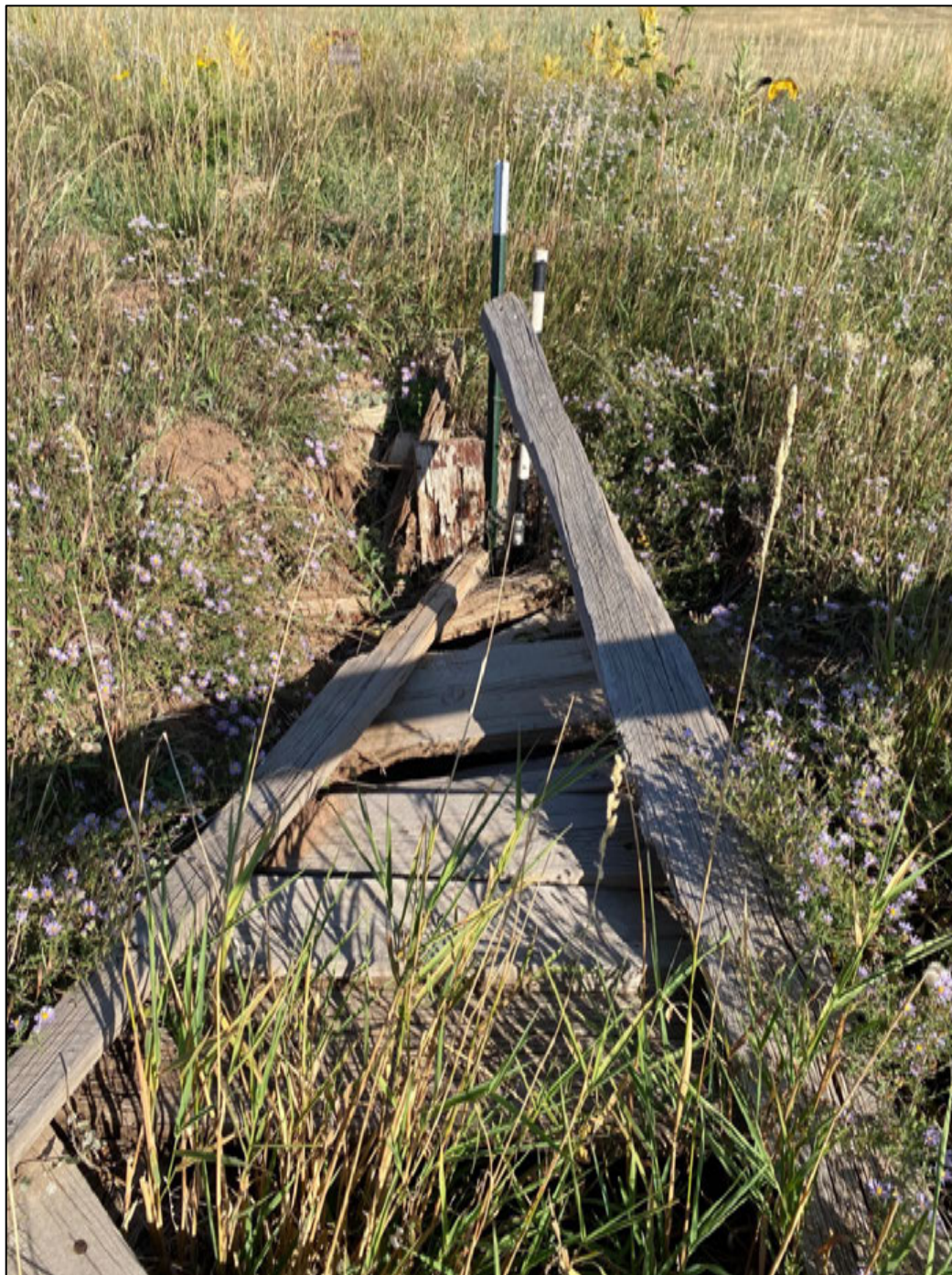
Figure 39. Closeup of the western face of the culvert and the boarded over stilling chute in Feature 8. View to the east.
