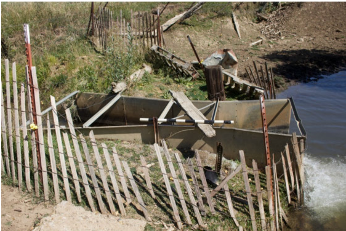
Image Number 5679 A photograph showing a closeup of Feature 5, the Ratliff and Root irrigation ditch Parshall Flume No. 2, facing west.
