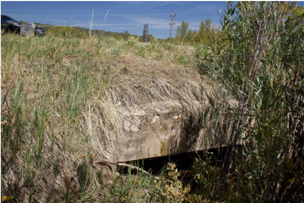
Image Number 5671 A photograph showing a closeup of concrete formed culvert under U.S. Highway 160 along the Ratliff and Root irrigation ditch, facing northeast.
