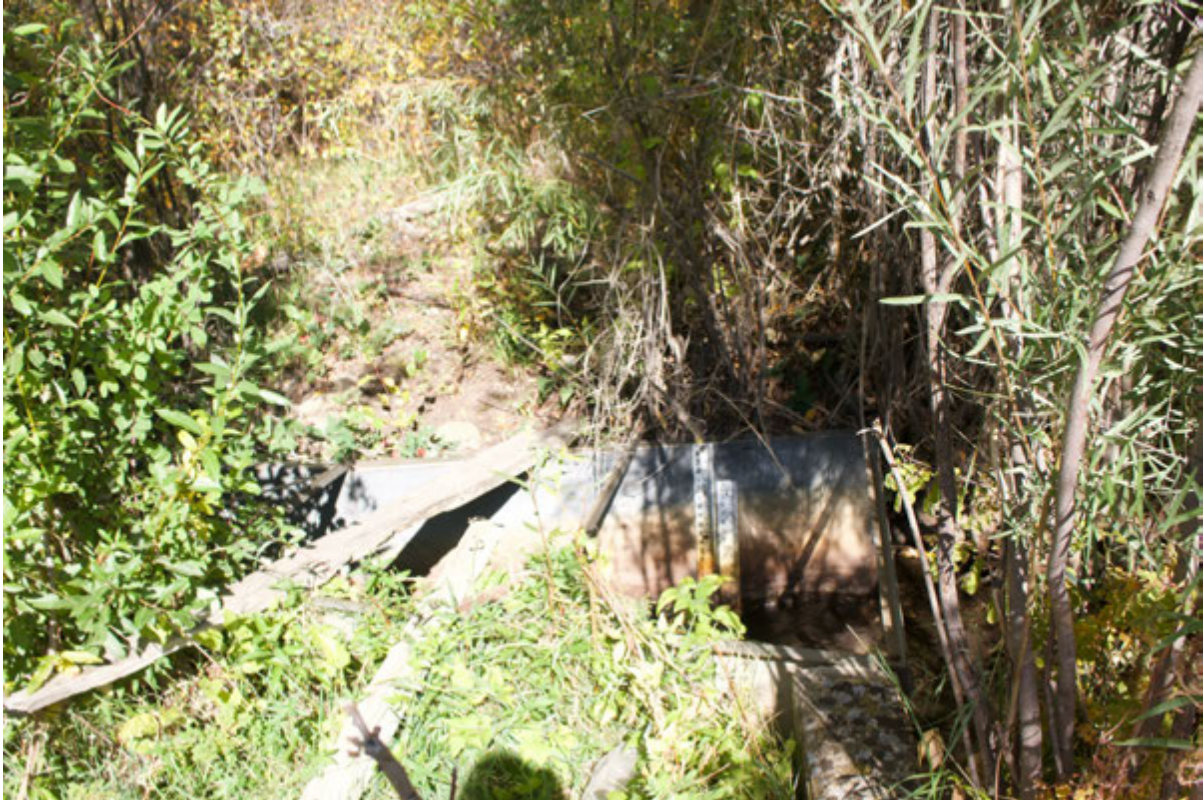
Image Number 5651 A photograph showing a closeup of Feature 3, the Ratliff and Root irrigation ditch Parshall Flume, facing north.
