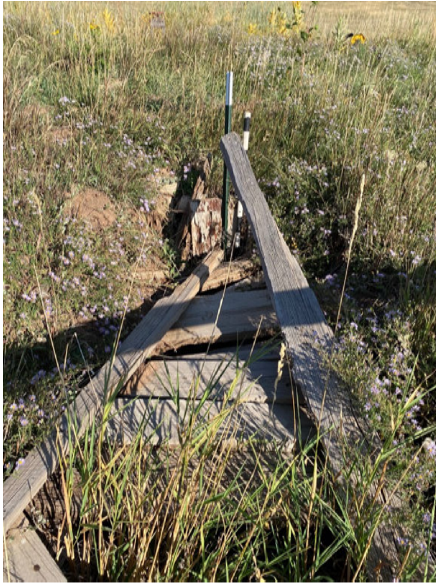
Image Number 5700 A photograph showing the west elevation of the concrete line culvert (covered by the board) in Feature 8, the Ratliff and Root irrigation ditch lateral ditch headgate. The boards in the foreground cover a stilling chute before a Parshall Flume, facing west.
