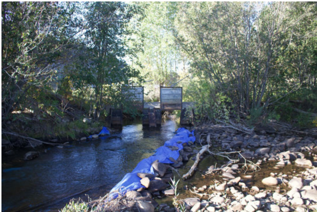
Image 5634 A photograph showing an overview of Feature 1, the Ratliff and Root irrigation ditch intake's Mancos River diversion berm and the intake gate in the background, facing south.
