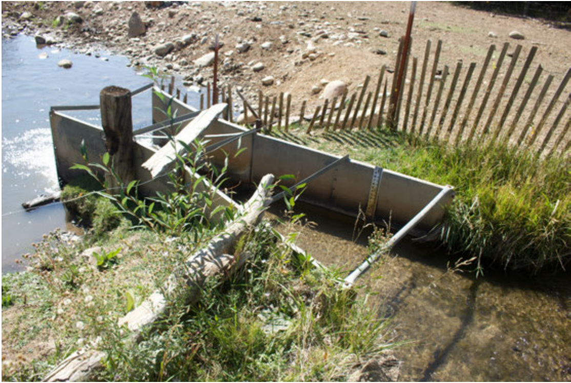
Image Number 5680 A photograph showing a closeup of Feature 5, the Ratliff and Root irrigation ditch Parshall Flume No. 2, facing southwest.
