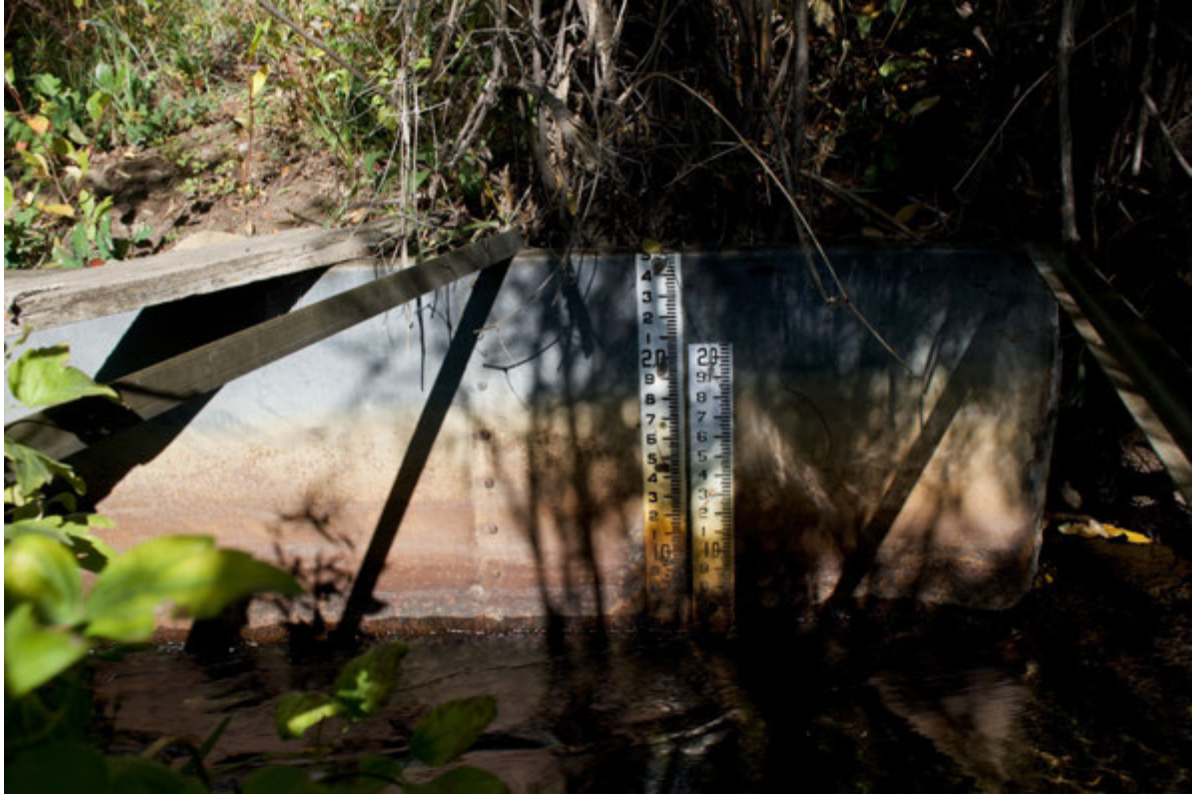
Image Number 5653 A photograph showing a closeup of Feature 3, the Ratliff and Root irrigation ditch Parshall Flume's flow rulers on the interior of the flume, facing north.
