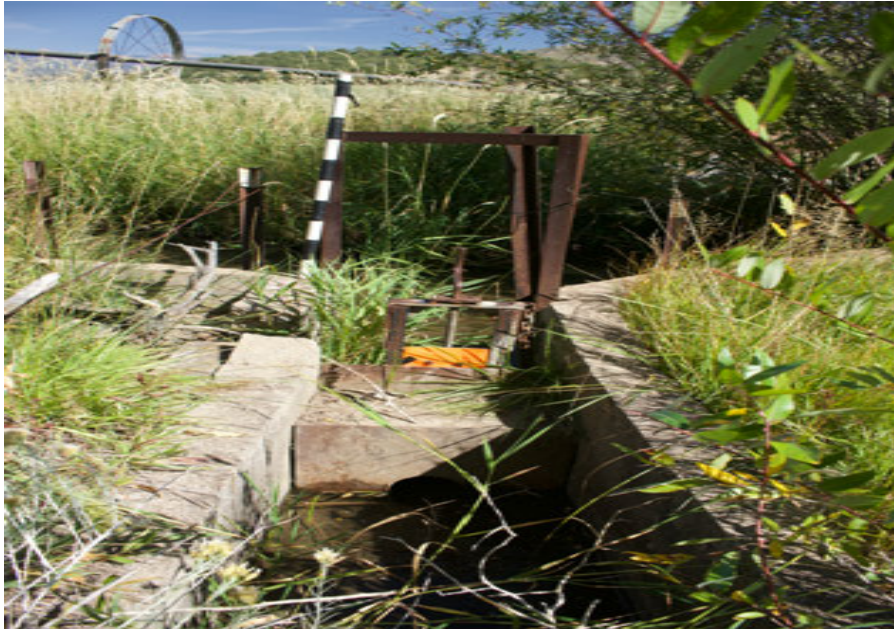
Figure 33. West elevation of lateral headgate in Feature 6.
