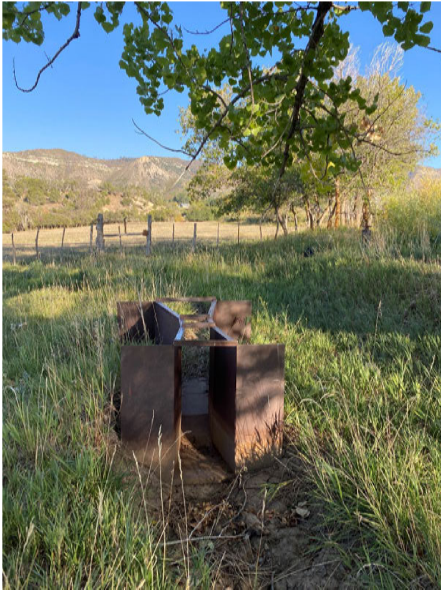
Image Number 5703 A photograph showing a closeup of the Parshall Flume in Feature 9 of the Ratliff and Root irrigation ditch, facing east.
