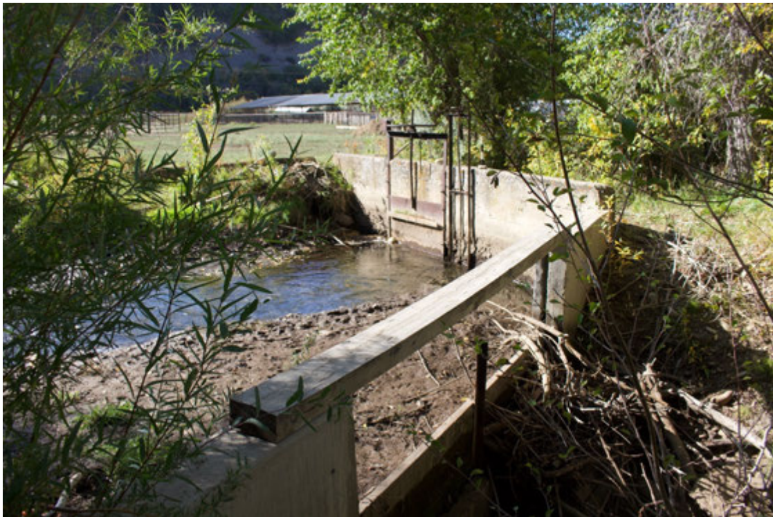
Image Number 5650 A photograph showing an overview of Feature 2, the Ratliff and Root irrigation ditch main headgates with Feature 1, the Ratliff and Root irrigation ditch's main intake in the background and Feature 2's overflow gate in the foreground, facing south.
