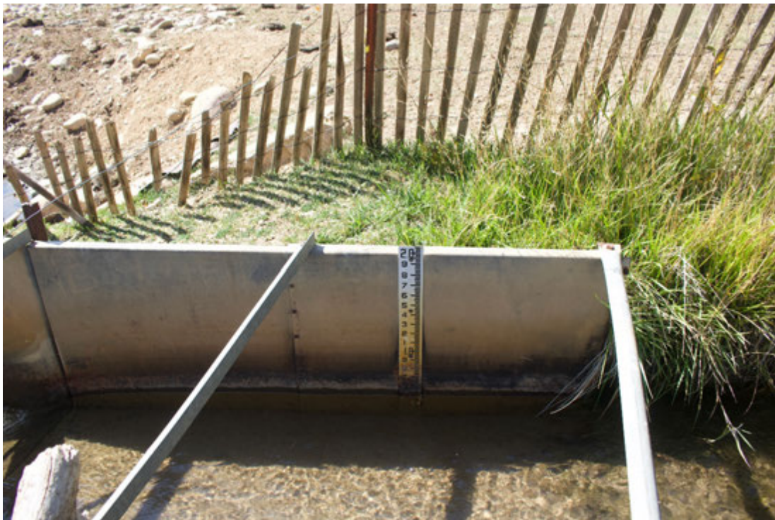
Image Number 5681 A photograph showing a closeup of Feature 5, the Ratliff and Root irrigation ditch Parshall Flume No. 2 water flow gauge, facing west.
