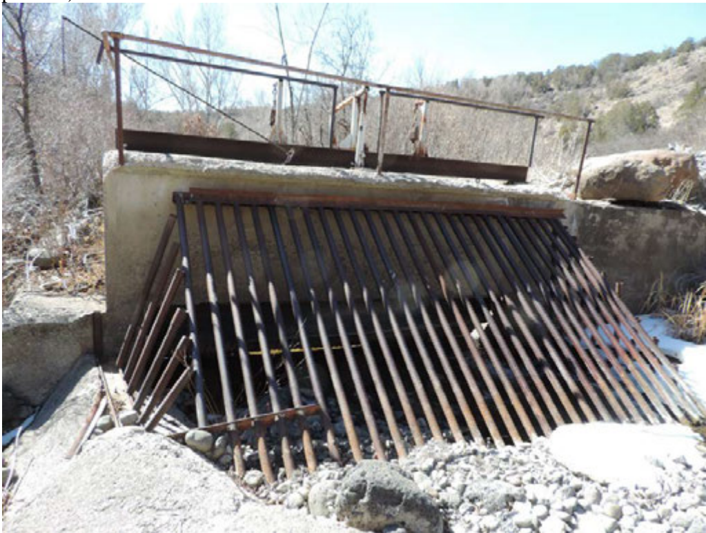
Figure 97: View south across the iron-pipe grate that prevents debris from entering the Leroux Creek Ditch channel, 5DT2005.3 (FAC Digital FMC Exp. 1888).
