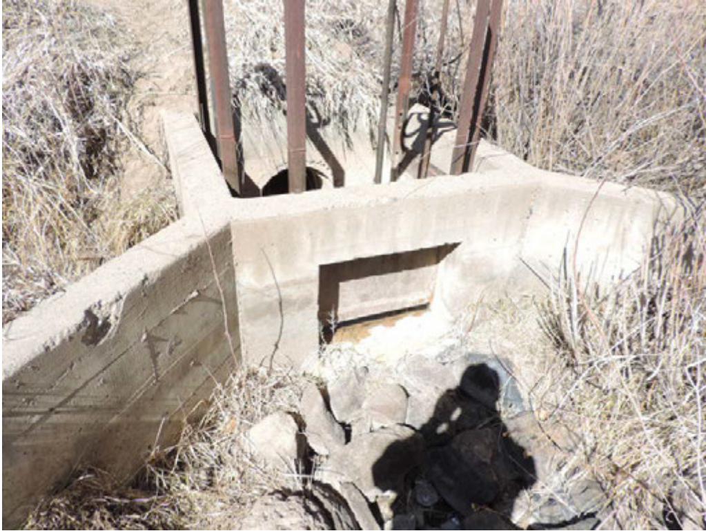
Figure 60: Close-up view of the gate controlling water flow at the tri-part structure of Feature 8, 5DT1277.4 (FAC Digital FMC Exp. 1930).
