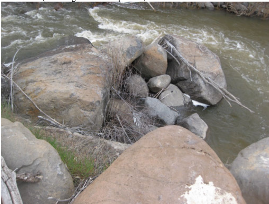
Figure 99: View north across boulder riprap designed to reduce the channel of Leroux Creek before entering the primary diversion area, 5DT2005.3 (FAC Digital FMC Exp. 3583).
