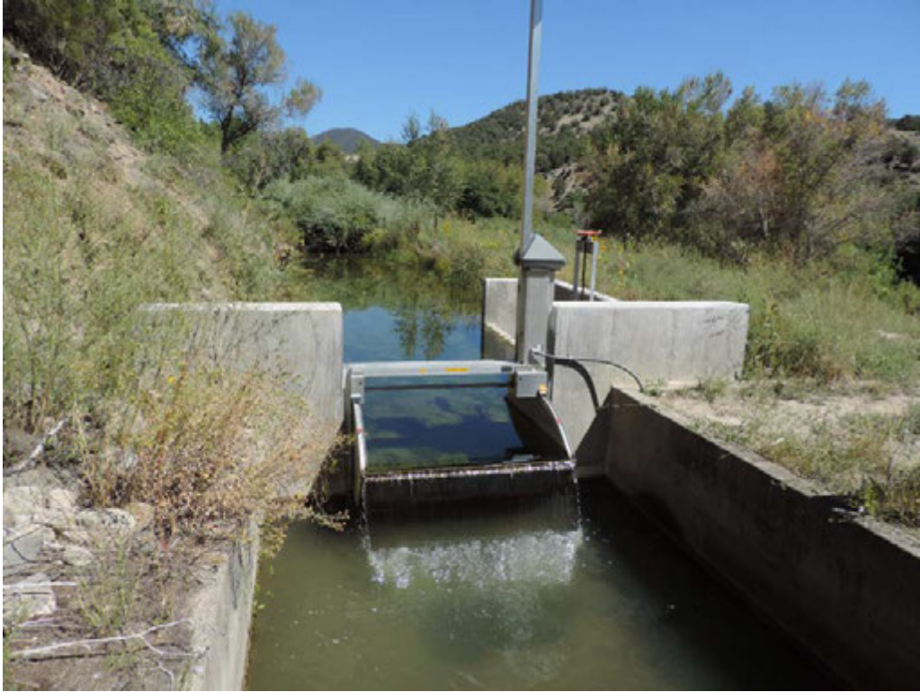
Figure 16: View north at the measuring weir at the point that the Leroux Creek Ditch (5DT2005.3) feeds into the Fire Mountain Canal segment 5DT1277.4 (FAC Digital FMC Exp. 1347).
