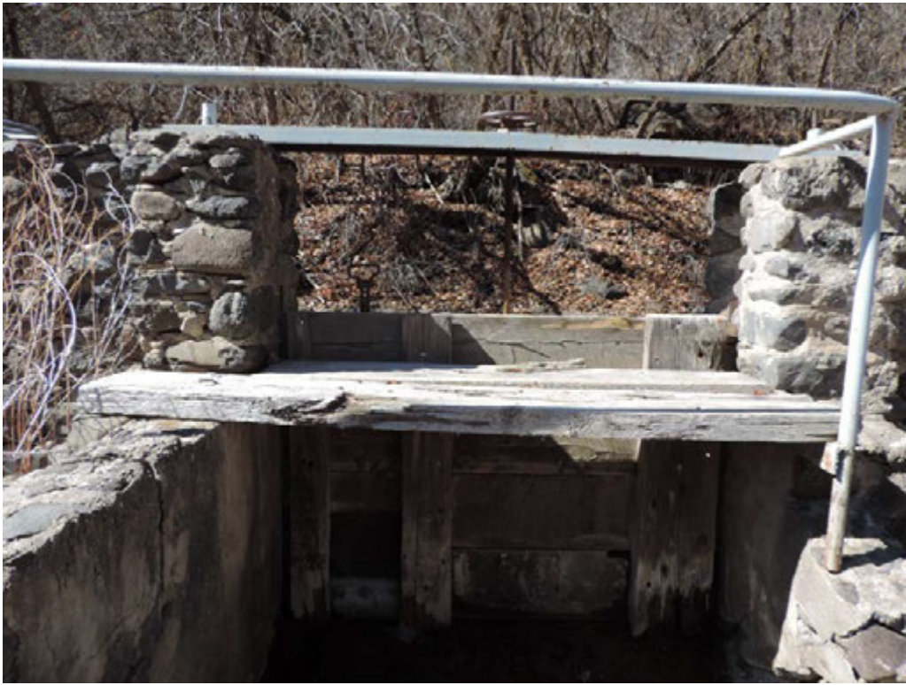
Figure 105: Close-up of the overflow gate of Feature 2, 5DT2005.3 (FAC Digital FMC Exp. 1908).
