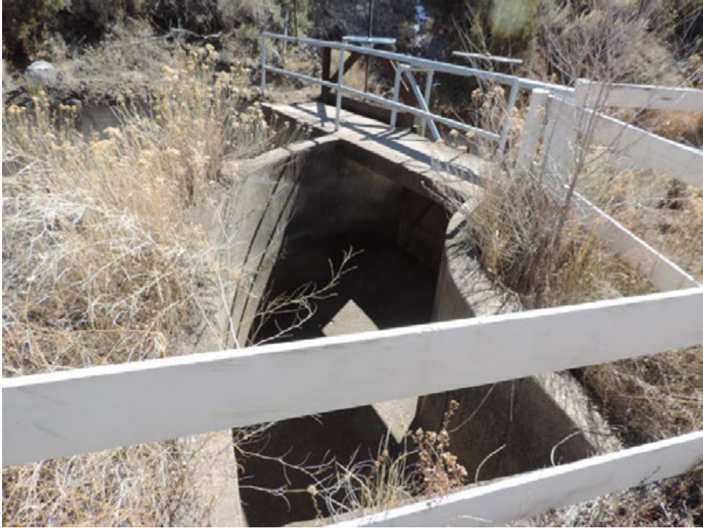
Figure 14: View down at the siphon channel of Feature 1a of the Fire Mountain Canal segment 5DT1277.4 (FAC Digital FMC Exp. 1857).
