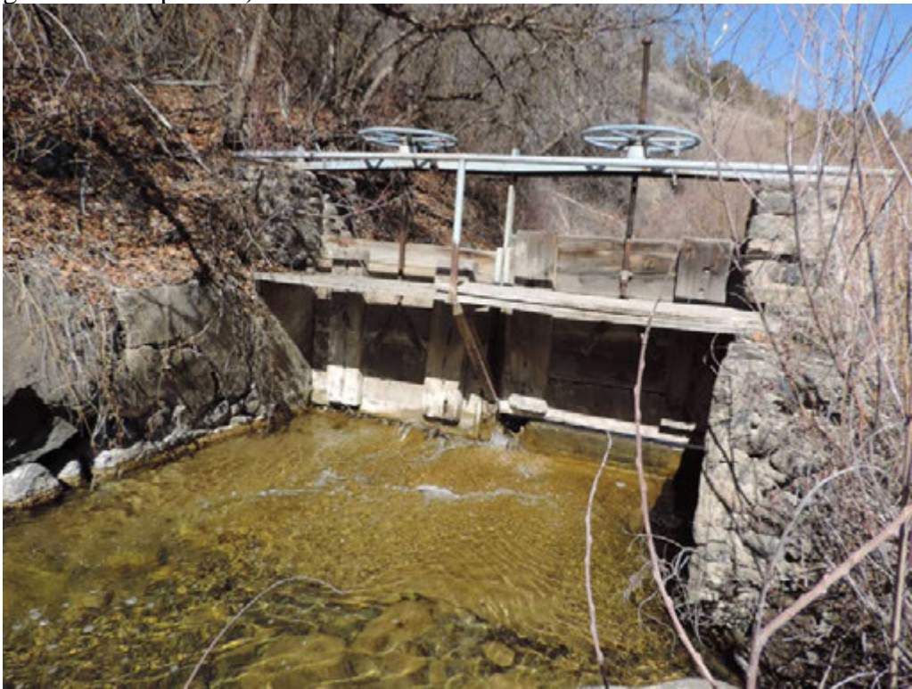
Figure 104: View north across the water flow control gates of Feature 2, 5DT2005.3 (FAC Digital FMC Exp. 1904).
