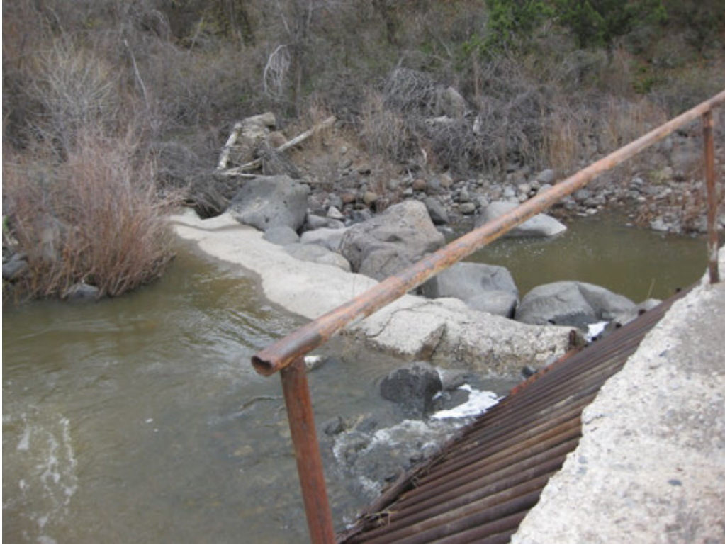
Figure 92: View northeast across the concrete and boulder riprap dam, 5DT2005.3 (FAC Digital FMC Exp. 3587).
