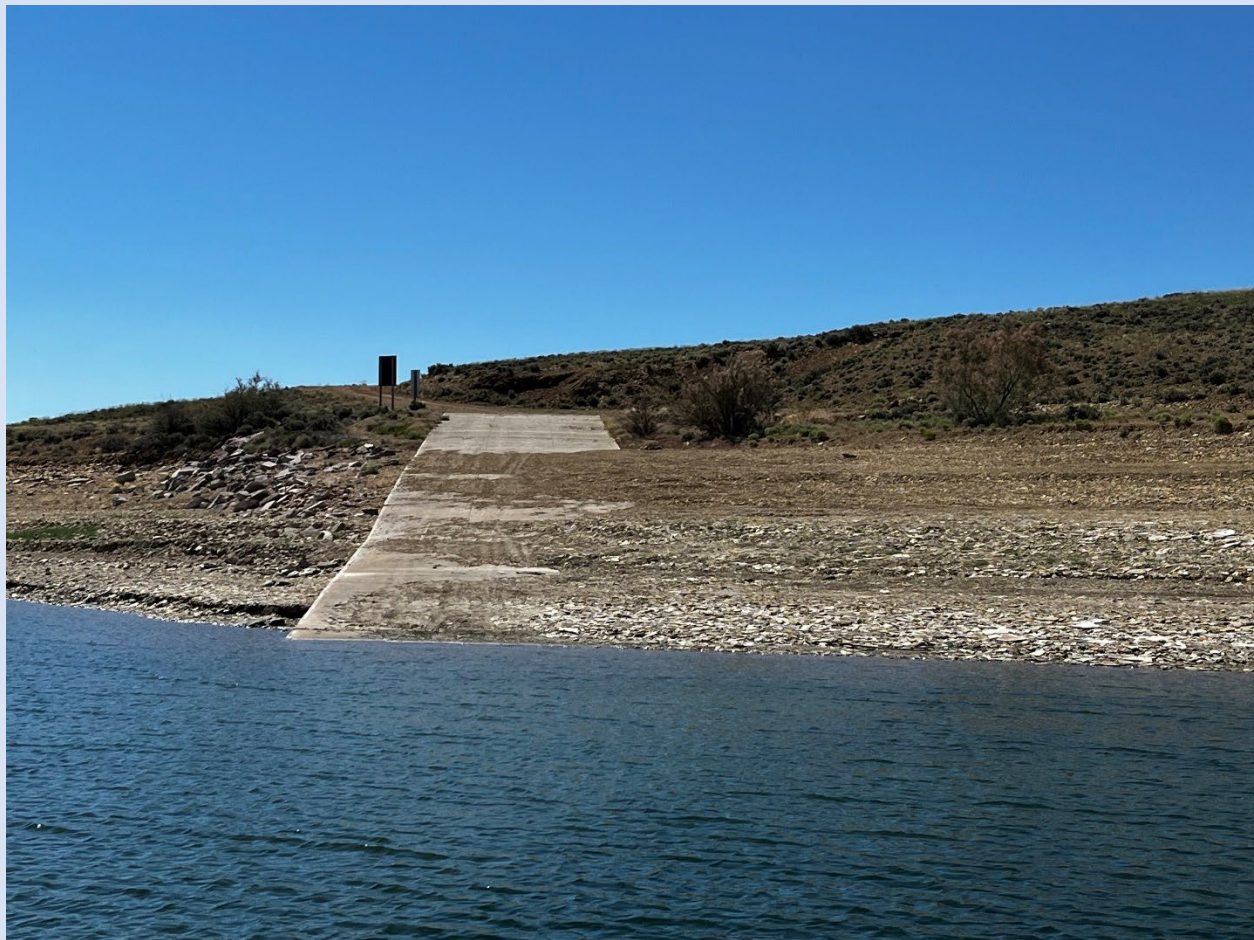
Figure 23. 2022 survey photograph showing sediments and rocks across the ramp face
