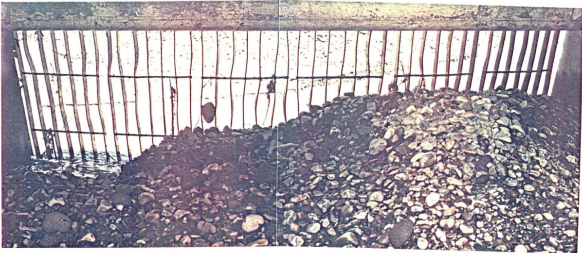
Photograph No. 5 - San Juan-Chama Project - Blanco Diversion Dam - View from inside structure of original trashrack and accumulated rock. Note rock along right is nearly to top of trashrack. Photo by R. Ochs August 26, 1980
