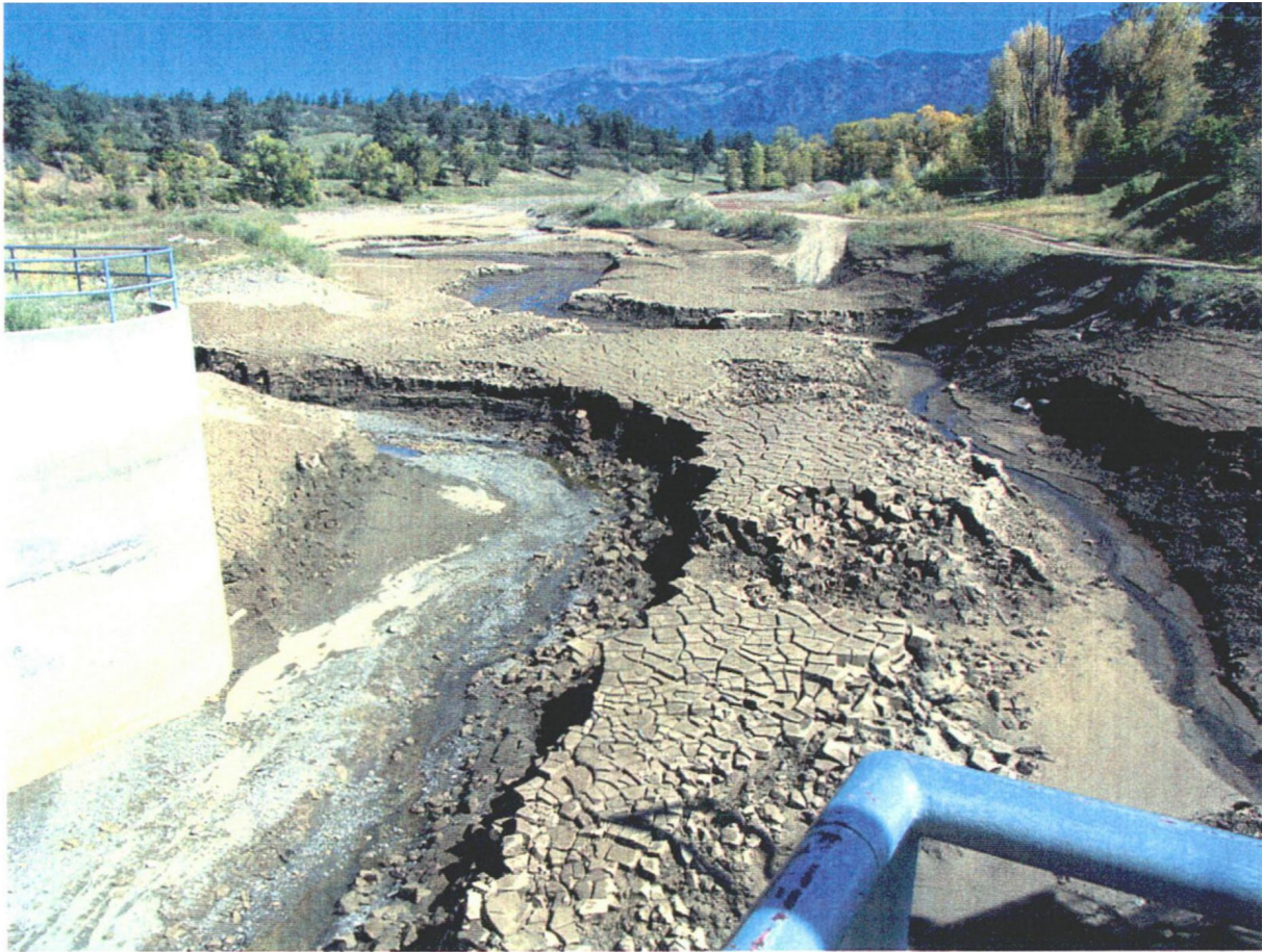
Photograph No. 36. Oso Diversion Dam – Upstream View of excess sediment buildup. Photograph Date 01/03/07 by: A. Vigil
