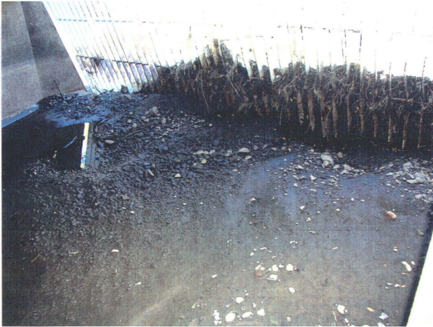
Photograph No. 14. Blanco Diversion Dam – Inside forebay. Note sedimentation buildup. Photograph Date 10/03/07 by: A. Vigil
