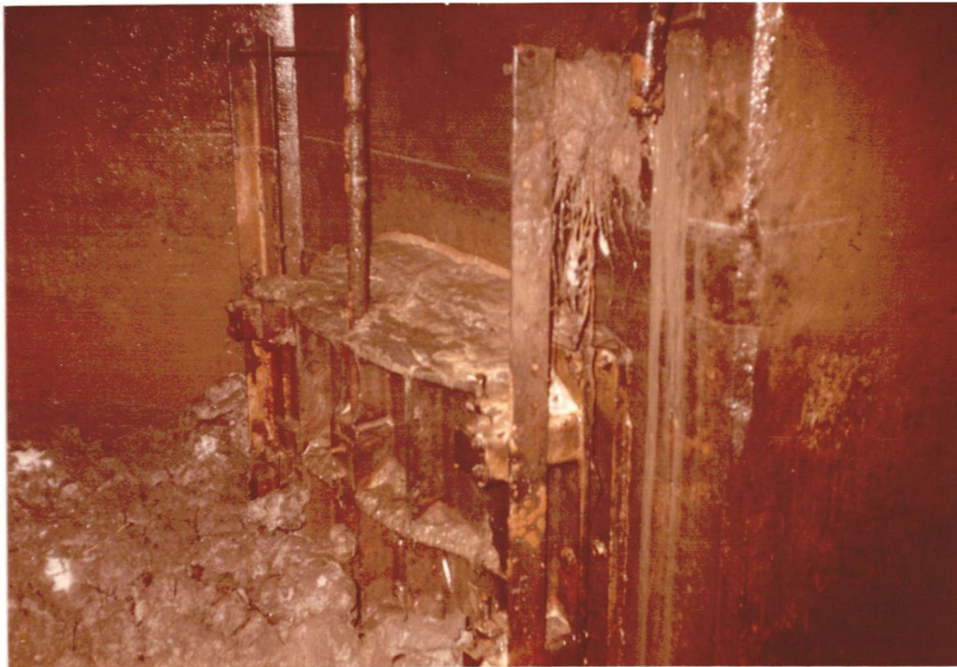
Figure 4.—Low flow diversion slide gate blocked by rocks (October 18, 1994).
