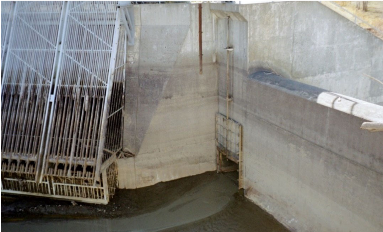
Figure 13.—Upstream facing side of Oso Dam showing sluiceway and gate, as well as headworks trashrack. Dam forebay is behind this trashrack. A portion of the headworks sill can also be seen.
