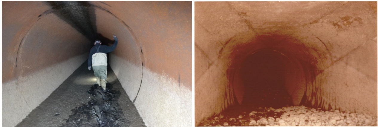
Figure 9.—Oso Siphon showing fine material deposition (left) and large size material at Oso Siphon outlet (right).
