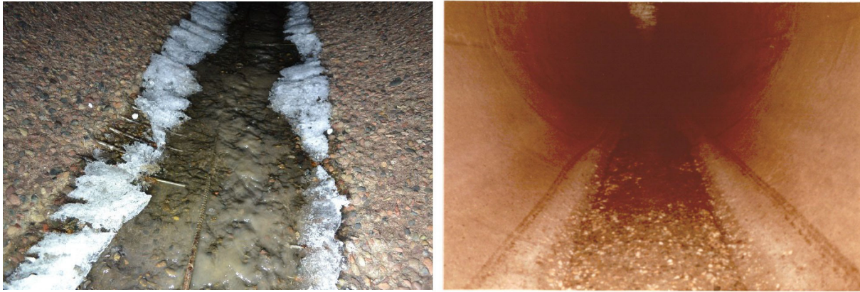
Figure 7.—Tunnel invert erosion at the edges of the repaired patch, (right) Oso Tunnel 2022 inspection photos, and (left) Oso Tunnel concrete invert repair made in 1983 showing a small amount of erosion after one year of diversions.
