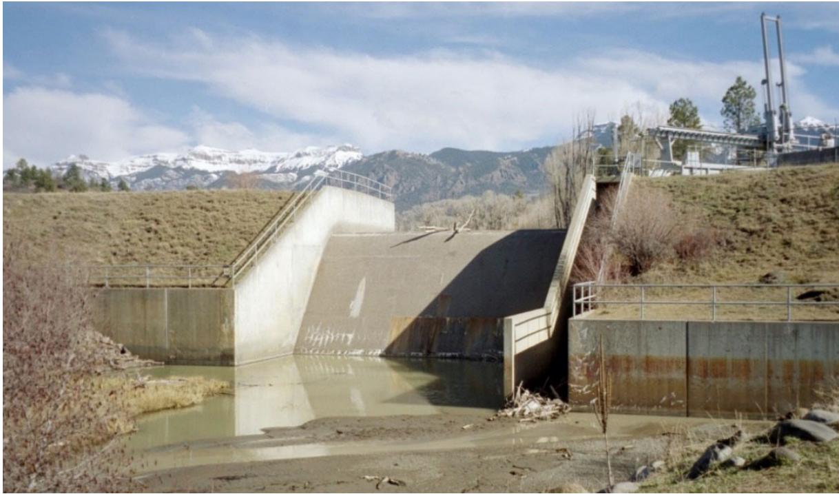
Figure 14.—Downstream side of Oso Dam showing spillway and sluiceway slot.
