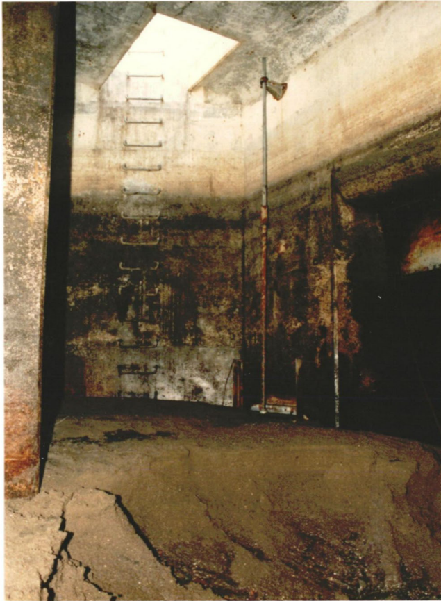
Photograph No. 74 - San Juan-Chama Project -- Oso Diversion Dam - View of the 36- by 36-inch low flow vertical slide gate located in the headwork to Oso Feeder Conduit.
