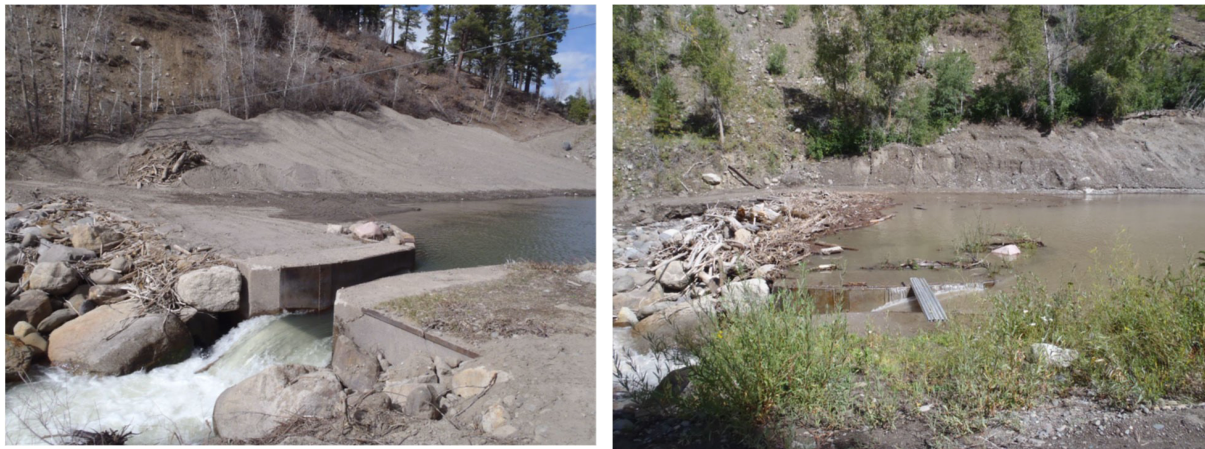
Figure 19.—Blanco River 4-foot Parshall Flume (left) and 60-foot weir at floodflow showing debris buildup (right). (photo by CODWR).
