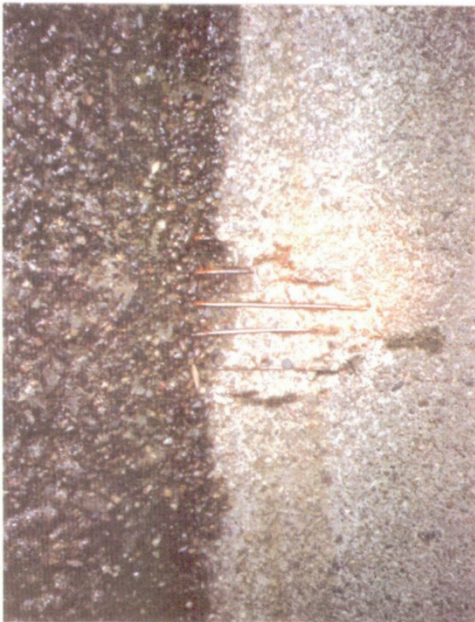
CN465-528-1855 Station 736+88. Photo shows exposed reinforcement in invert of Oso Siphon. Figure 18.
