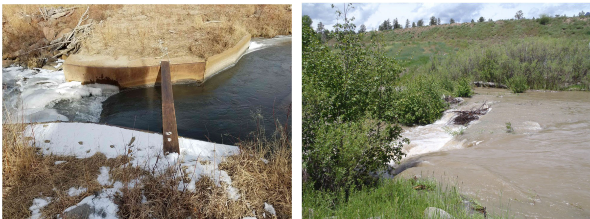
Figure 20.—Navajo River bypass gage 8-foot Parshall flume (left) and 60-foot weir at floodflow (photo by CODWR).
