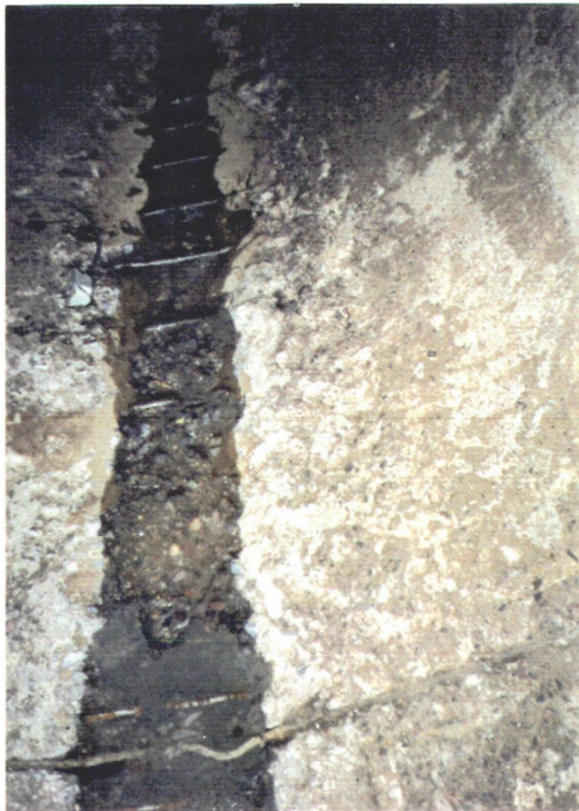
Photograph No. 5 - San Juan-Chama Project - Blanco Diversion Dam - View from inside structure of original trashrack and accumulated rock. Note rock along right is nearly to top of trashrack. Photo by R. Ochs August 26, 1980
