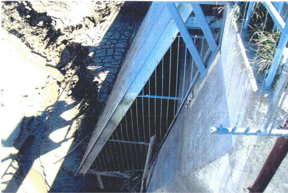
Photograph No. 38. Oso Diversion Dam – View of sediment buildup on Trash-Rack System. Photograph Date 10/03/07 by: A. Vigil
