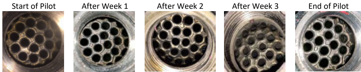
Figure 6: SaltMaker Pilot Heat Exchanger Inspections
