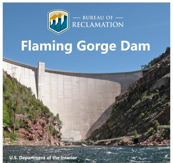
Flaming Gorge Dam rises 502 feet above the bedrock of the Green River, 32 miles south of the Utah-Wyoming border, and forms the Flaming Gorge Reservoir that extends 91 miles north into Wyoming. The reservoir has a total capacity of nearly 3.8 million acre-feet and, at the full capacity elevation of 6,040 feet above sea level, the reservoir has a surface area of 42,020 acres and 375 miles of shoreline.
