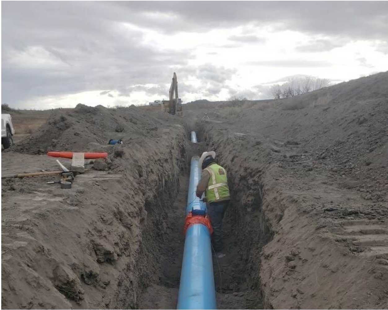
Photograph 1. Example of the pipeline installation process for an irrigation lateral in the Uncompahgre Valley, completed in 2020 (David Bridges, UVWUA).
