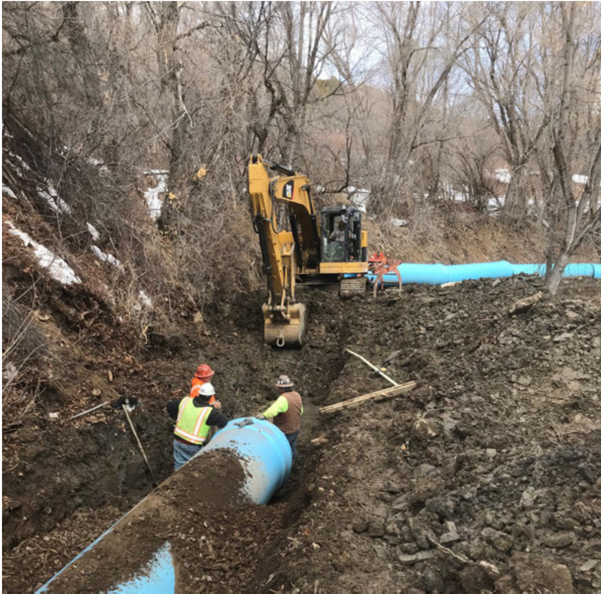
Photograph 1. Example of the pipeline installation process on the upper Needle Rock Ditch in the area just below the headgate, completed in 2019. (Applegate Group, Inc.)
