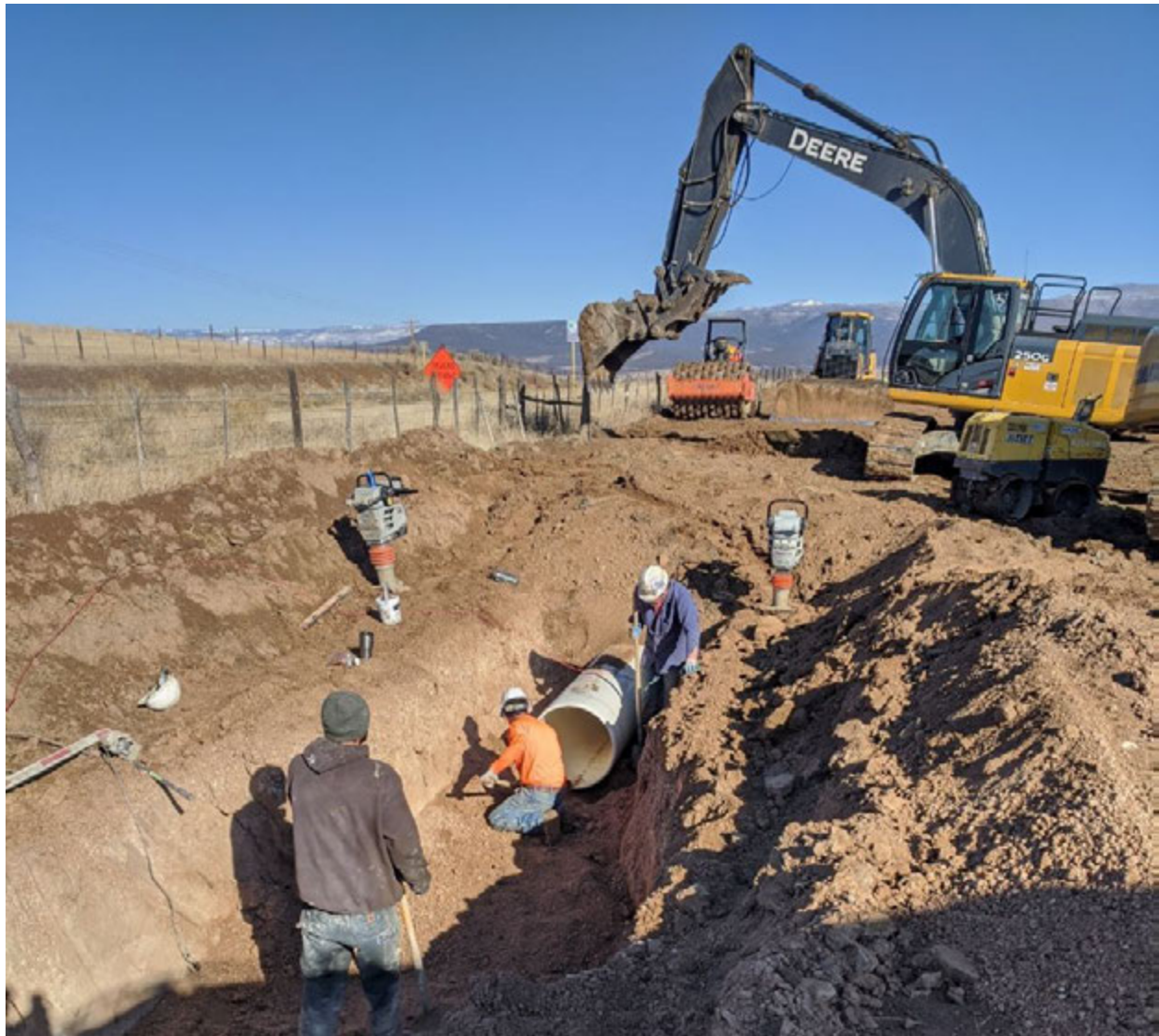
Photograph 1. Example of the pipeline installation process on a different CCDC salinity control piping project. (Harward Engineering/Marcel Orton)
