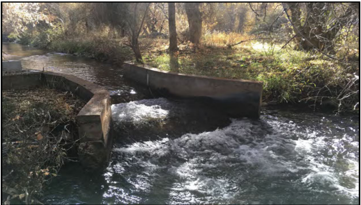
Photo 2. The existing Parshall flume near the head of the South Bench Canal.
