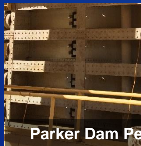
CP System on Pump Columns in Sump, 1990
