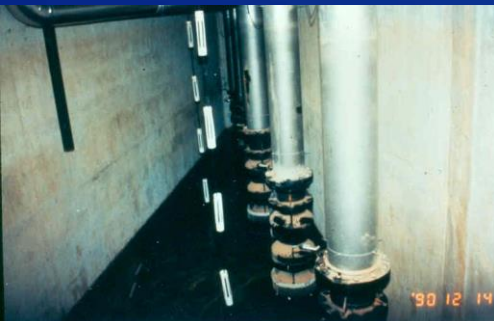
CP System on Pump Columns in Sump, 1990
