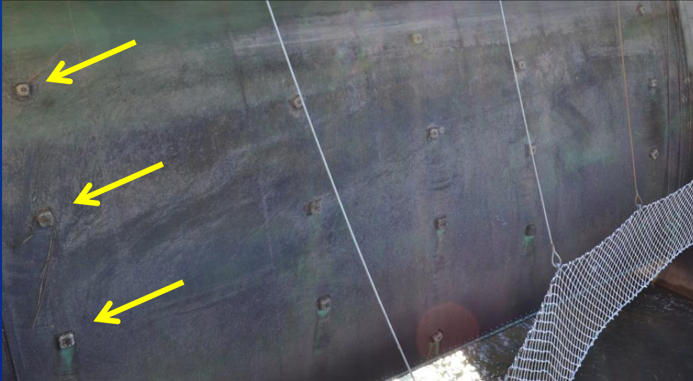
New vs. Old Mg Anode
