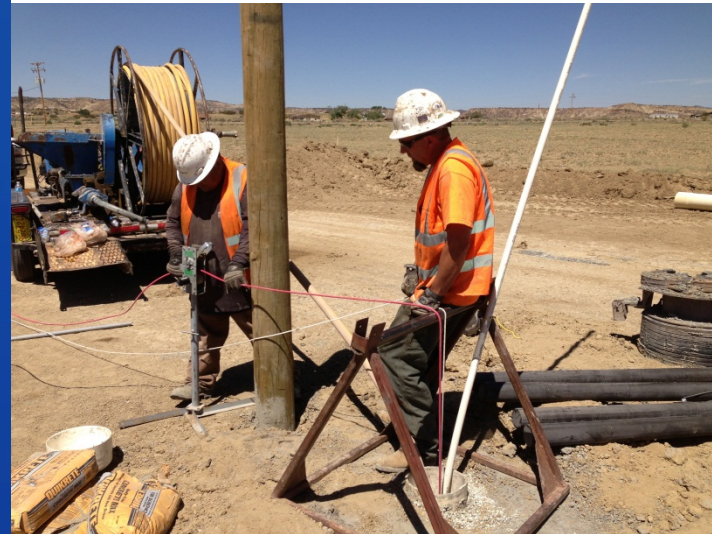
Graphite anodes in deep well IC system
