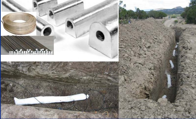
Mg Anodes in GA horizontal bed
