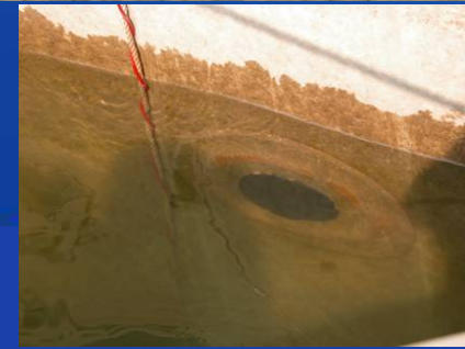
Mixed Metal Oxide Disk Anode
