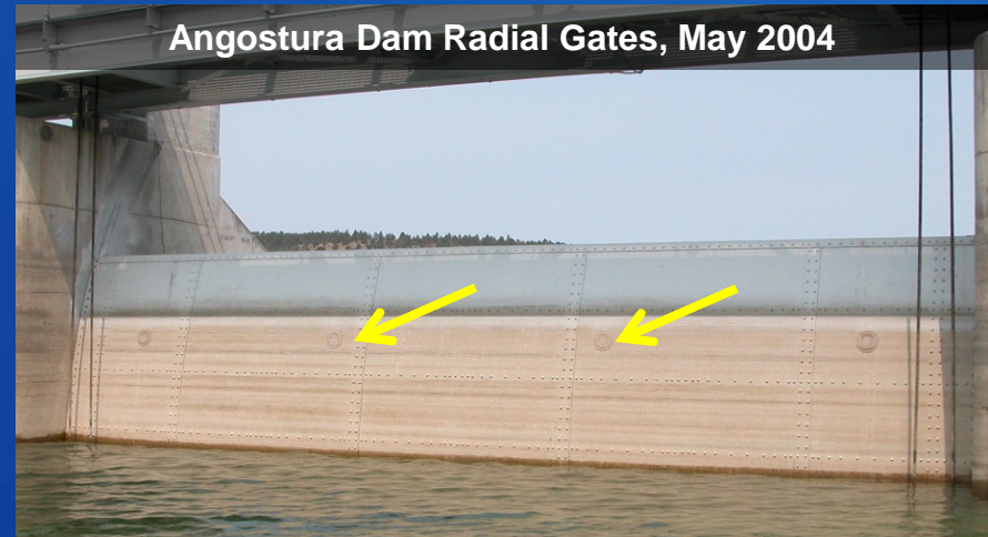
Mixed Metal Oxide Disk Anode
