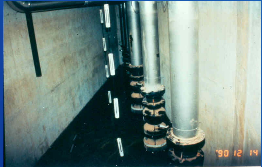
CP System on Pump Columns in Sump
