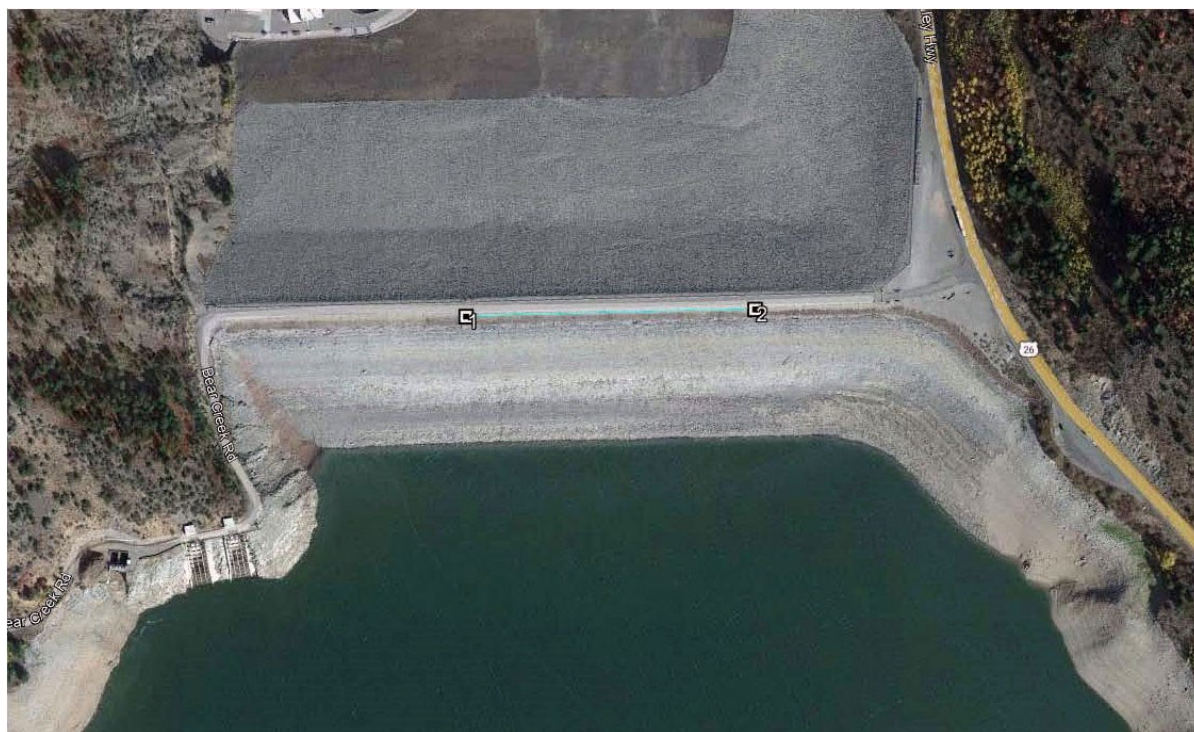
Points #1 and #2, Monitoring Point (24+00 and 6+00).
