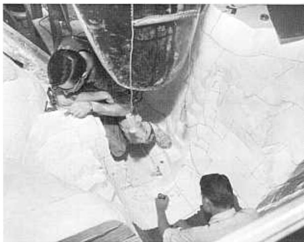
Figure 7.—Shaping abutments and foundation—Morrow Point model.
