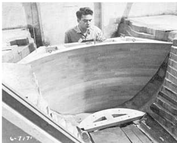
Figure 8. —Upstream and lower sections of downstream form in place—Glen Canyon model.
