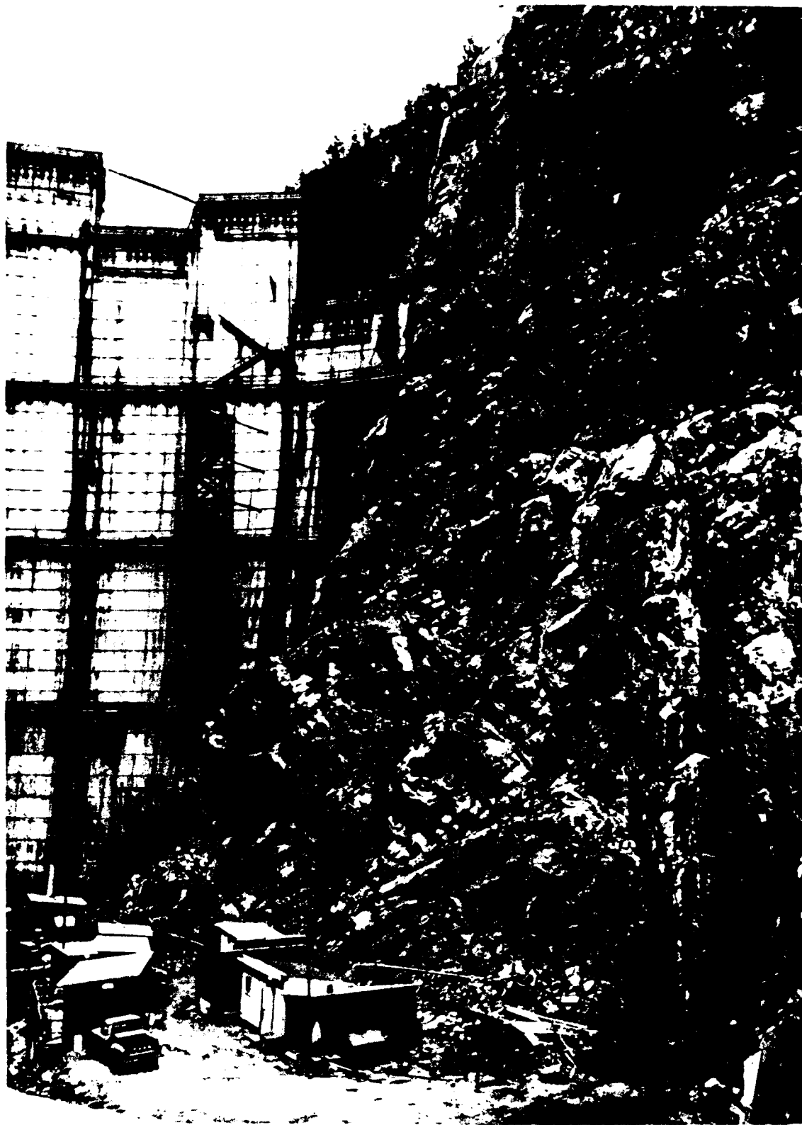
P622B-427-3698 NA--Curecanti Unit - Morrow Point Dam - Colorado-- View of the powerplant open cut area above the downstream portal of draft tube No. 1. Grout which leaked out above draft tube No. 1 during the foudation grouting of Block 4 at Elev. 6956+ can be seen in the right center of the picture. Johnson-MK, Spec. DC-5915. 8-31-66
