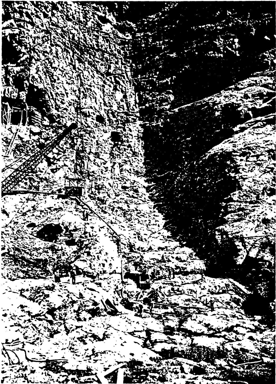
P622B-427-3081 NA---Curecanti Unit---Morrow Point Dam---Colorado View of the right keyway after excavation has been completed. Grouting is in progress. 8-4-65
