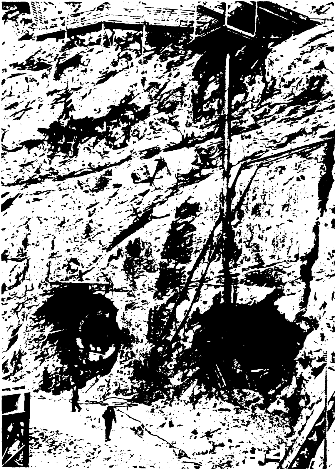
P622B-427-3977 NA--Curecanti Unit - Morrow Point Dam - Colorado Penstock: View of the upstream portal of the penstocks. The areas for the Intake Structure base slabs has been excavated and are being cleaned up. Bulkheads for winter protection are visible in both penstock tunnels. Johnson--M.K., Spec. No. DC-5915. 3-8-67
