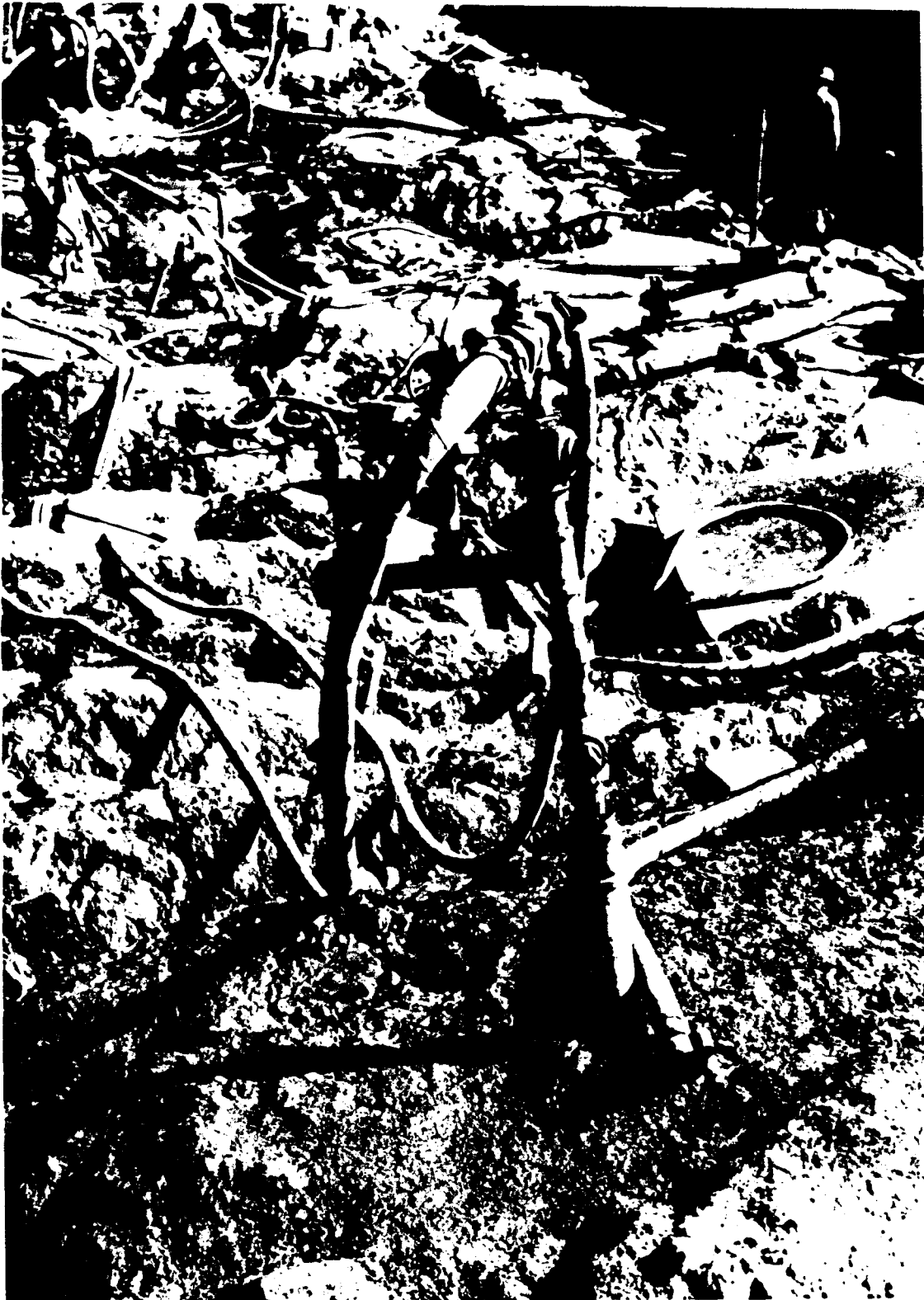
P622B-427-3100 NA--Curecanti Unit - Morrow Point Dam - Colorado-- Typical grouting manifold. Hole is being grouted from nipple. Johnson-MK, Specification No. DC-5915. 8-18-65
