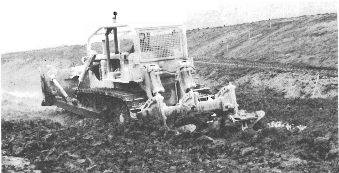
Figure 6. — Mixing quicklime with expansive clay. P801-D-80752
