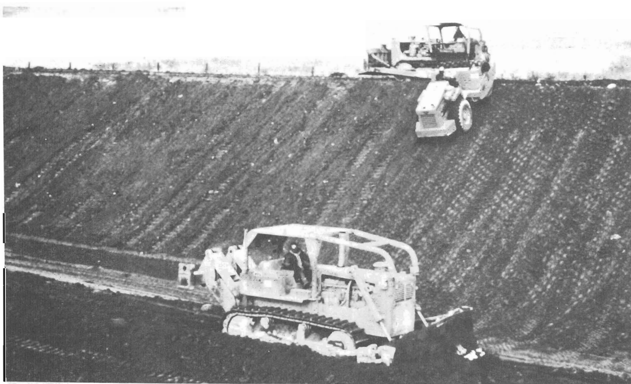
Figure 8. — Compaction of soil-lime canal lining. P801-D-80754
