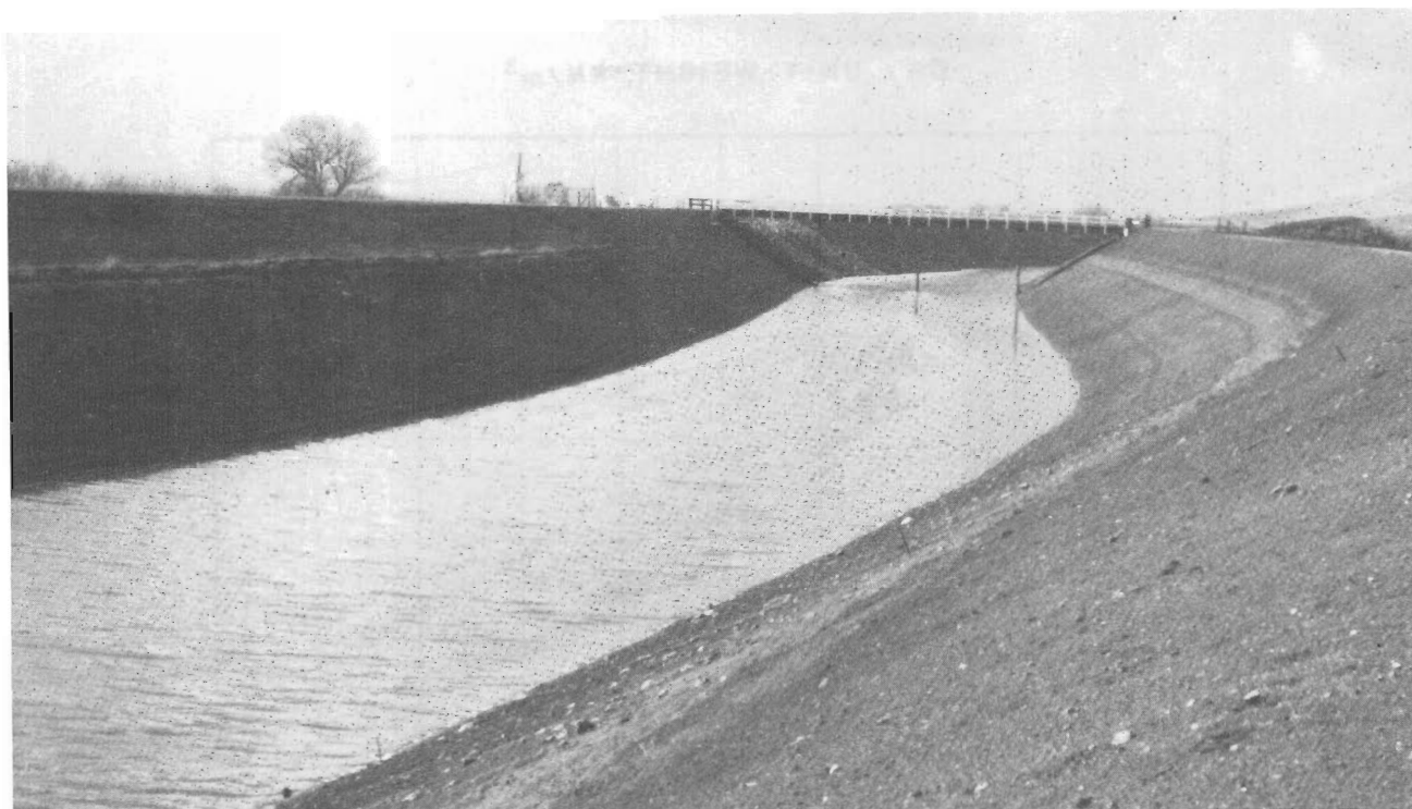
Figure 13. — Soil-lime lining on Friant-Kern Canal after 5 years of operation. P801-D-80755
