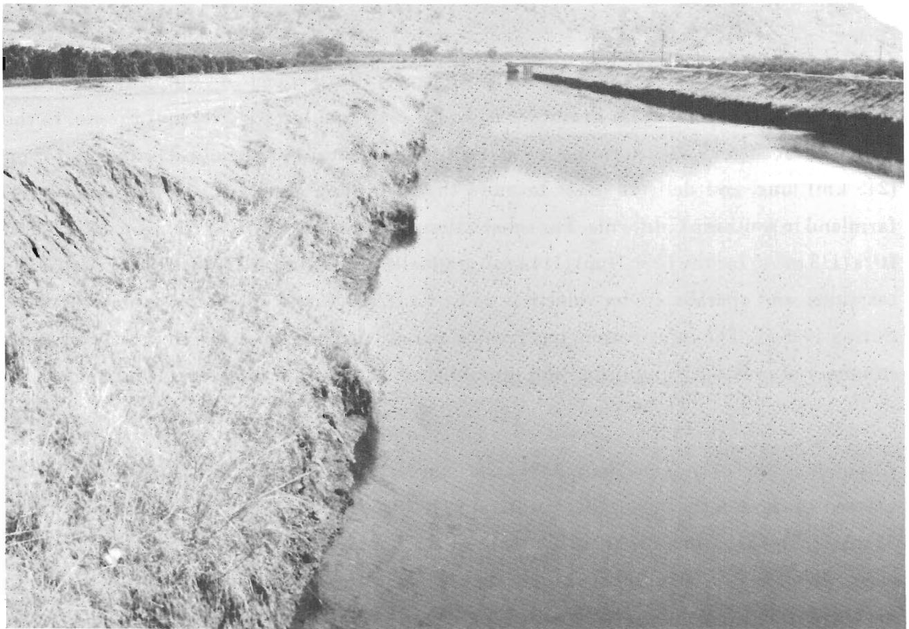
Figure 1. — Friant-Kern Canal prior to lime stabilization. Note slope failure along linings, P801-D-80750
