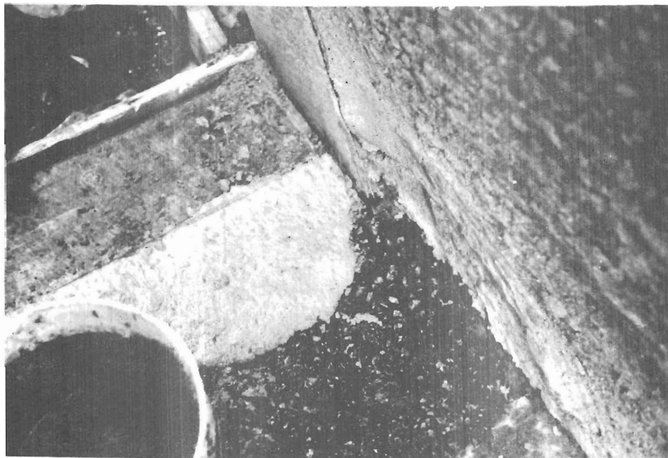
Polymer concrete mortar being applied downstream from sill plate.
