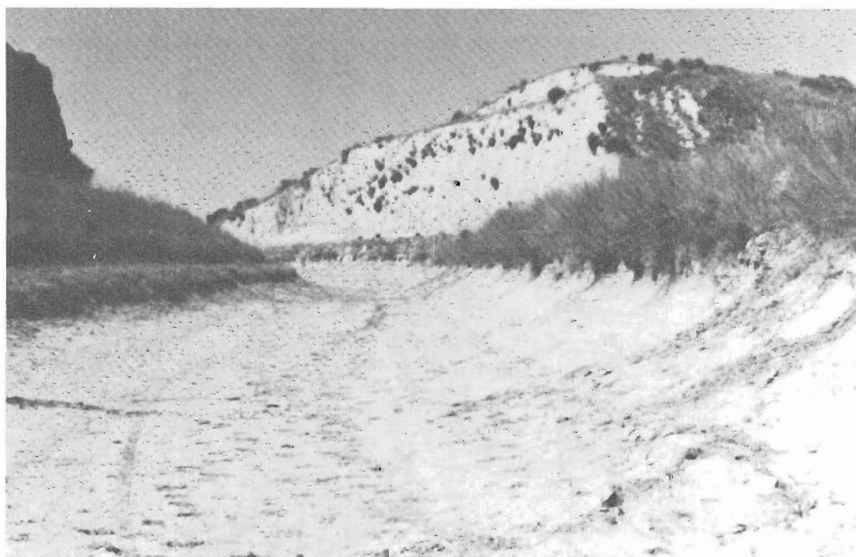
Figure 11. — Looking upstream at sampling location for 2.5 percent cement-modified soil lining at station 314+25. Treated bank on right and untreated bank on left. P801-D-80033.
