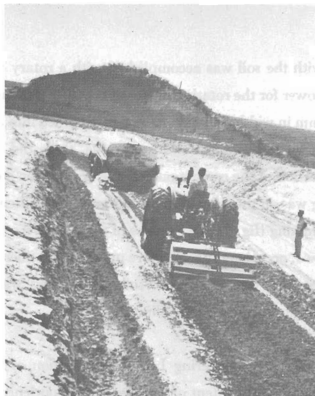
Figure 7. — Watering and mixing the soil and cement with a Seaman rotary tiller. July 1958. P801-D-80029.
