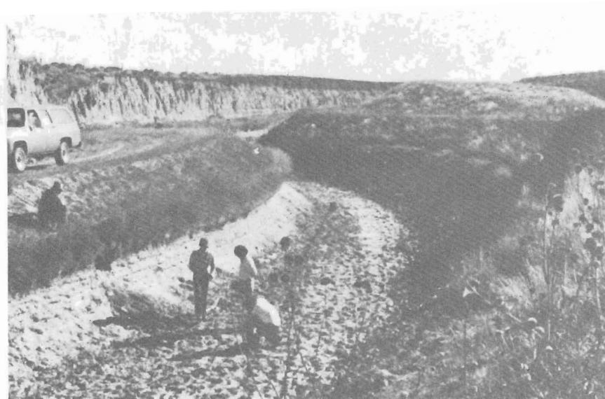
Figure 8. — Sampling location in 4.5 percent cement-modified reach on inside curve at station 299+82. Gravel has been added on the opposite, untreated bank to reduce erosion. P801-D-80030.
