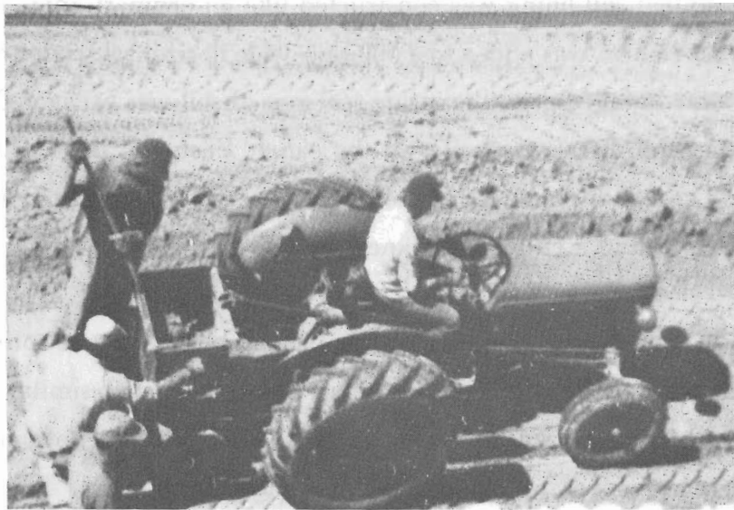
Figure 6. — Tractor-mounted, shop-made spreader for placing the 600-mm-wide strip of cement. July 1958. P801-D-80028.
